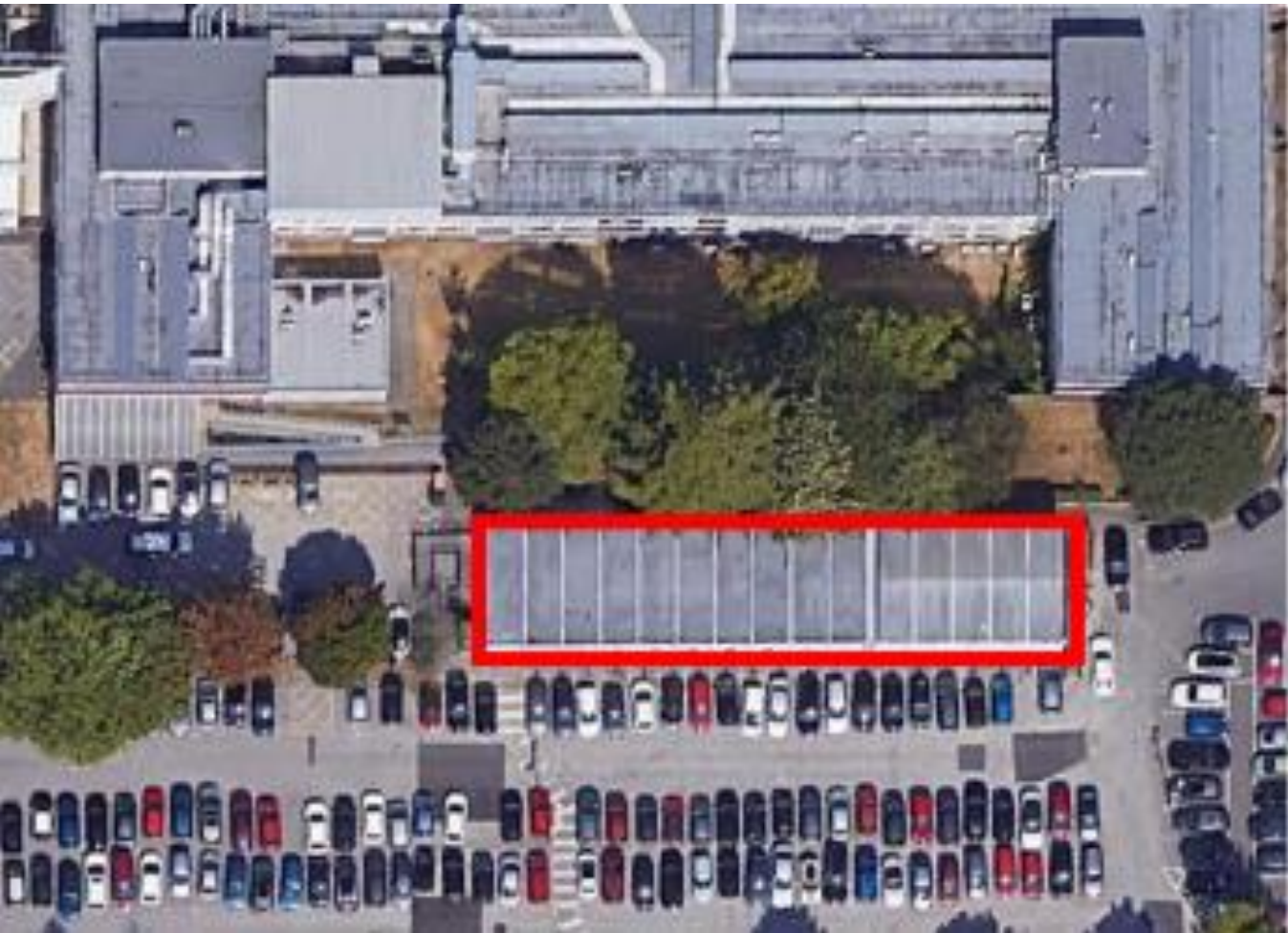
Figure 1.1 – Current South Block Annex building
