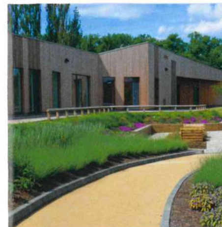
Timber vertical boarding
