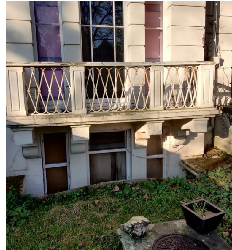
View from front garden down to Lower Ground Floor windows
