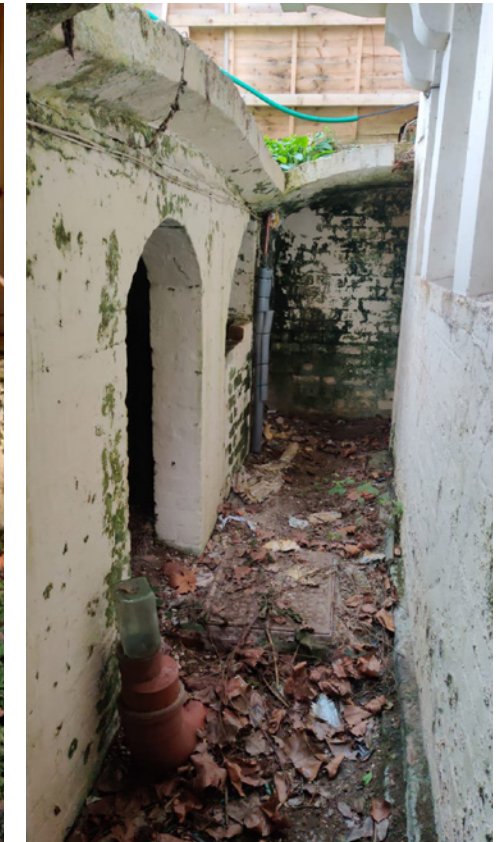
Lightwell vaults in front of windows
