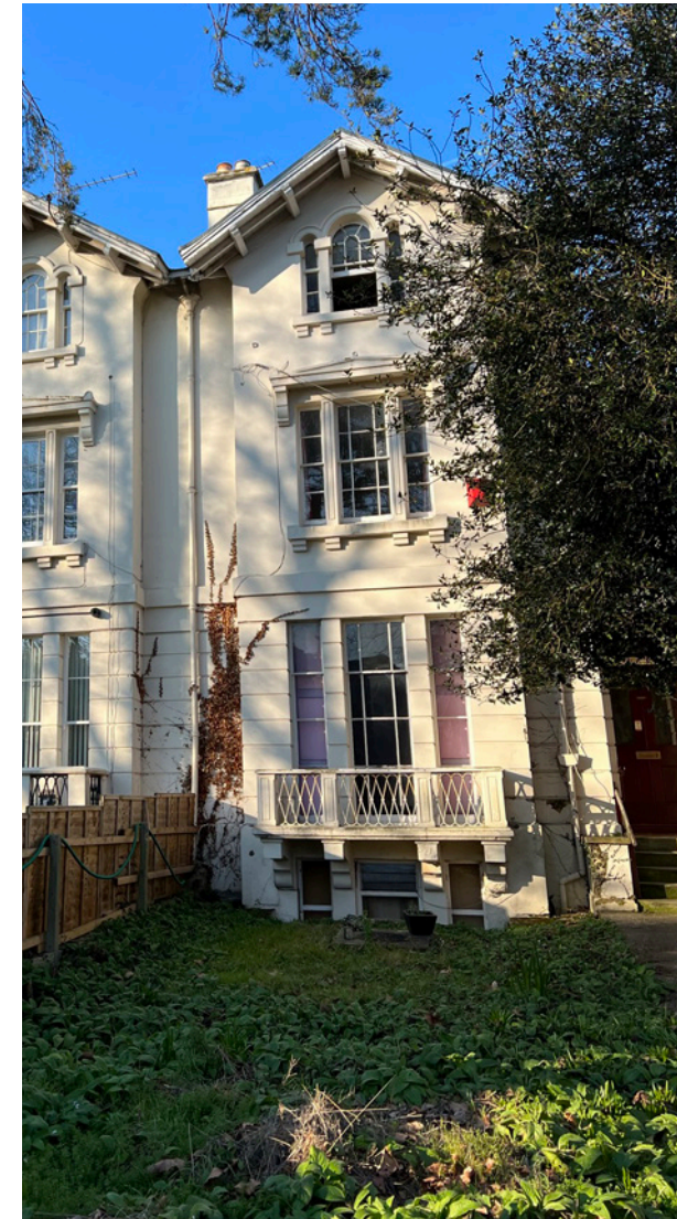
View of no. 83 & 85 from the front garden of no. 85
