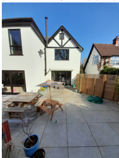
Site photo: rear elevation
