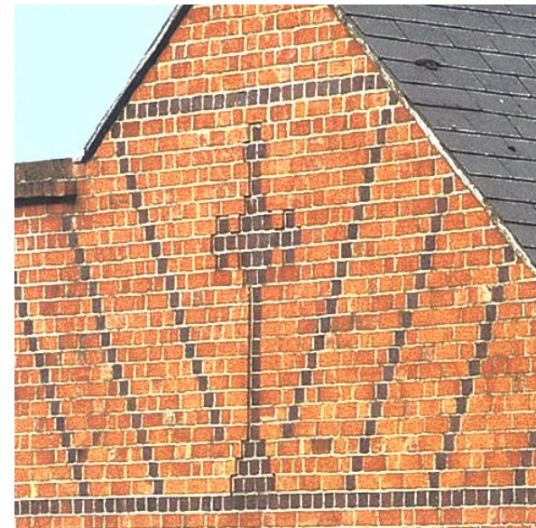
Stepped Crosses of Purple Bricks, River Rd
