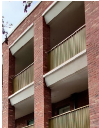
HTA Design - West Green Place Deck Access
