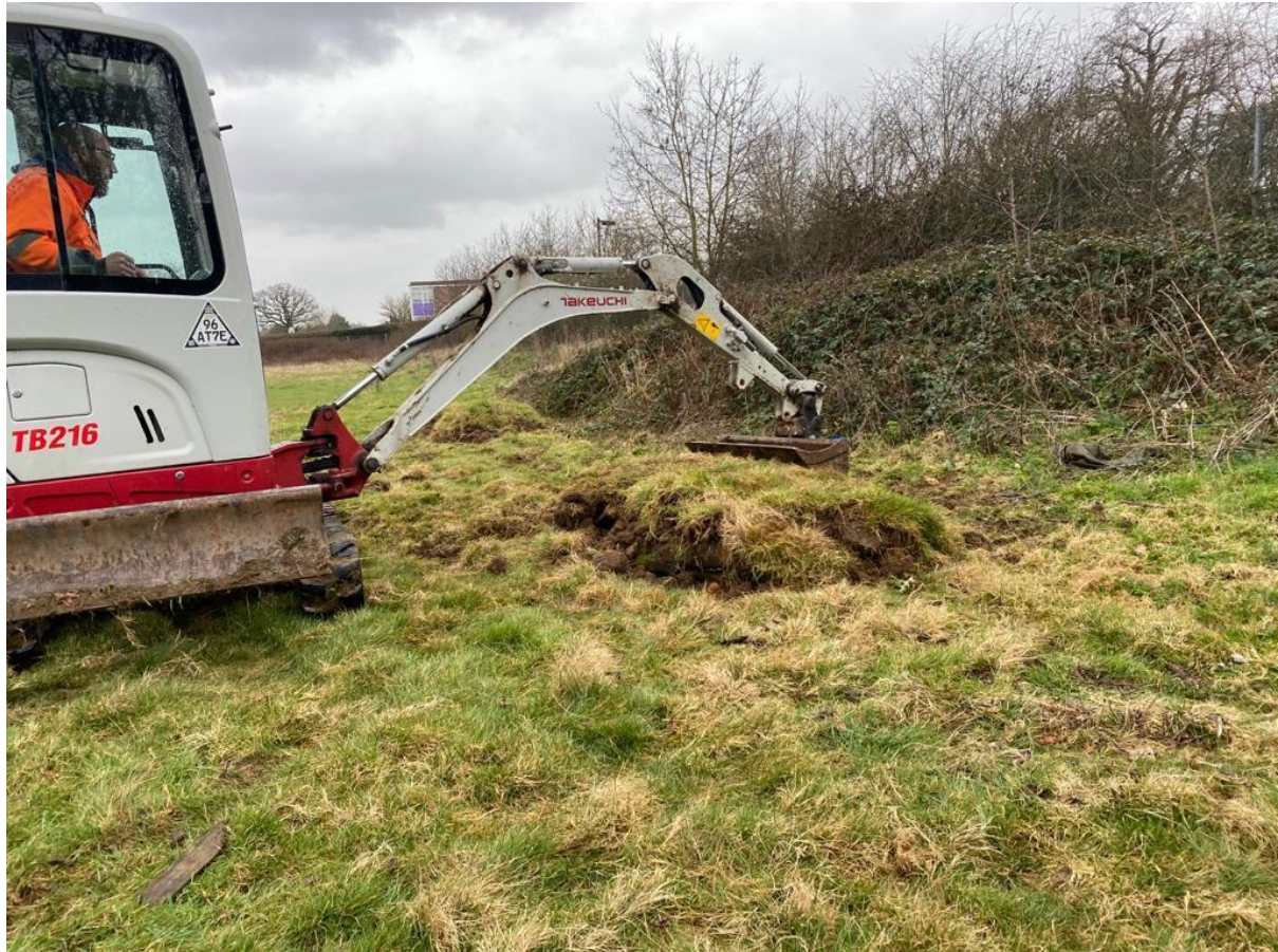
Figure 5. View of destructive search undertaken with a toothed bucket digger. Image produced Courtesy of GreenWays Countryside Management Ltd 2023.
