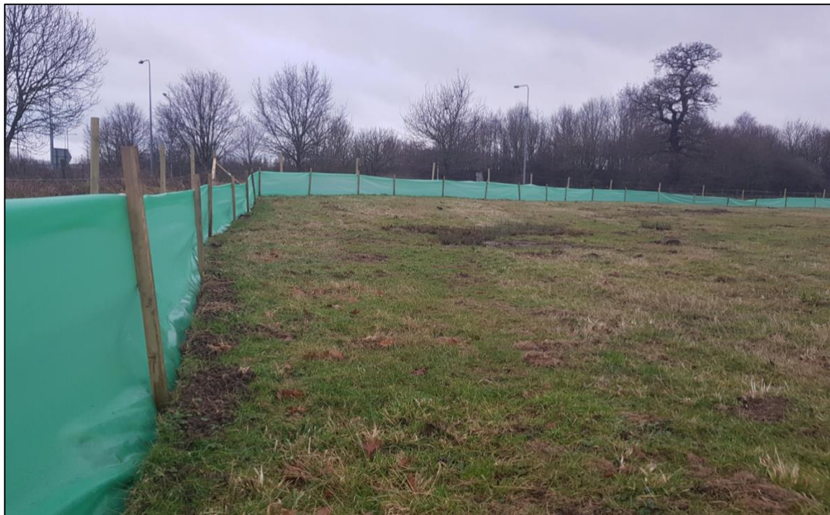
Figure 10. An example of the temporary fencing material that will be used.
