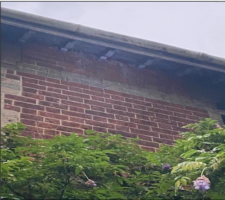
Plate 4: This image shows bird droppings along the wall plate of the main brick building (indicating recent bird nesting activity).
