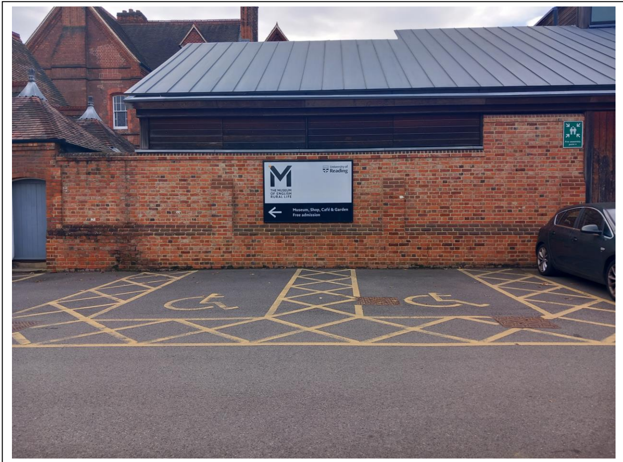
The end of the listed building is the brick pillar to the right of the door. The Museum of English Rural Life, London Road, Reading RG1. Photo illustrates wall to which the EV chargers will be mounted.
