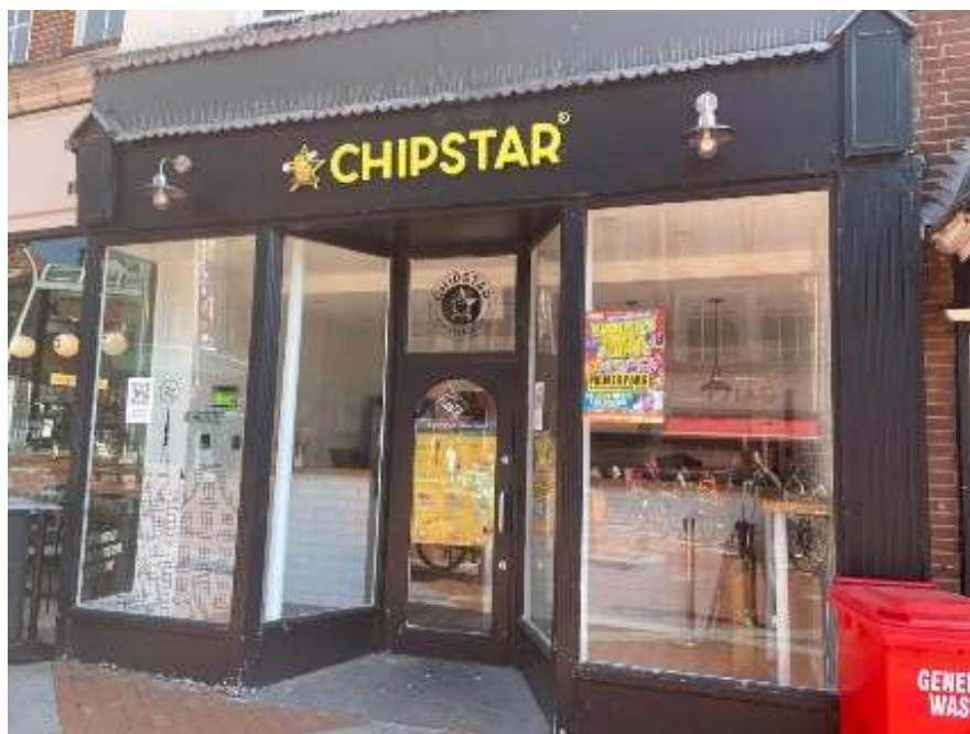
A photograph of the existing shop front.
