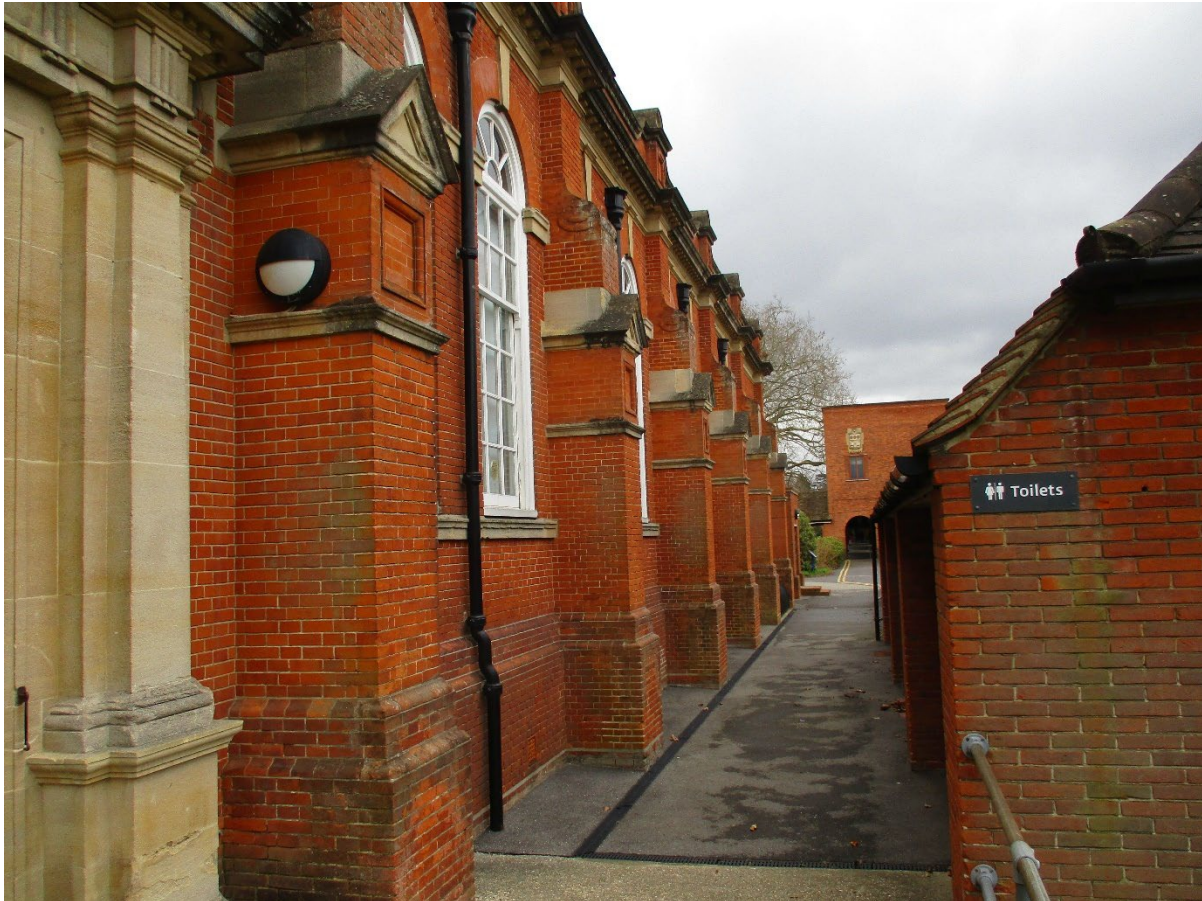
Disabled Toilet – Access must be always clear.
