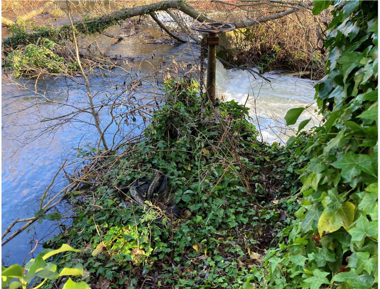
Photograph 2 - Weir Structure adjacent to the Site's northern boundary
