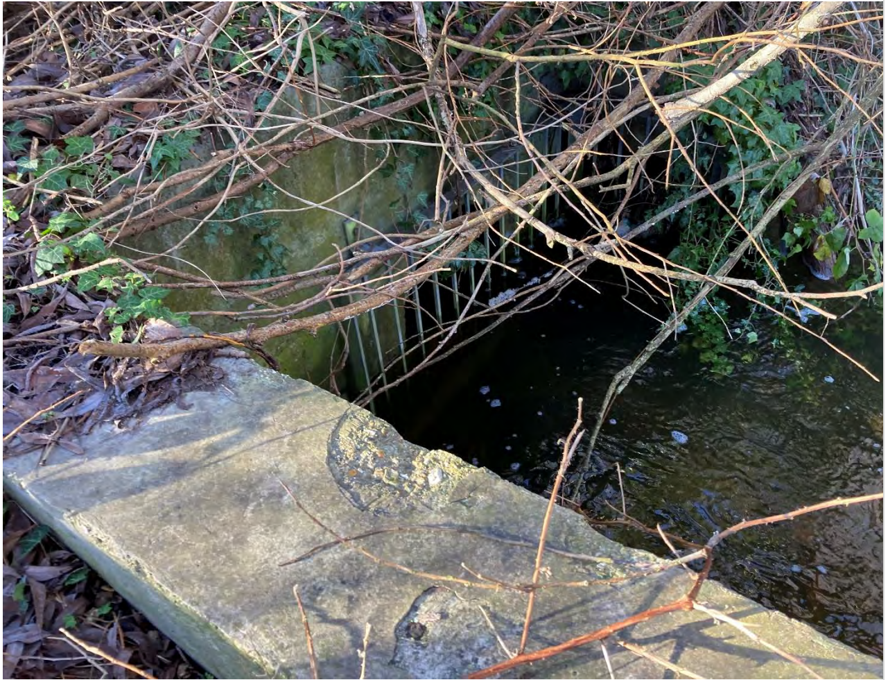
Photograph 1 - Storm Water drain outlet located to the north of the Site
