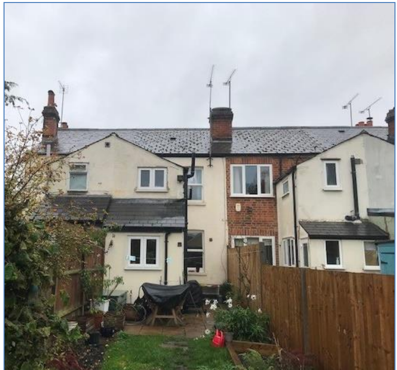
2. Rear of 38 and 40 Piggotts Road. Photo provided by the agent on 30/10/2020.
