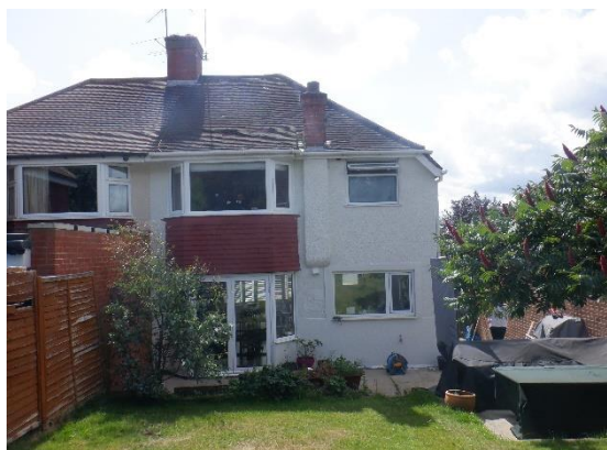
2. Rear of property viewed from the north.
