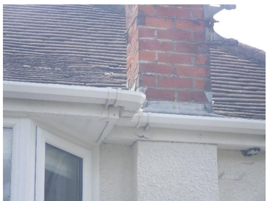
4. Tight lead flashing around the chimney.
