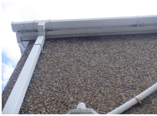
6. Soffits tight and sealed throughout.
