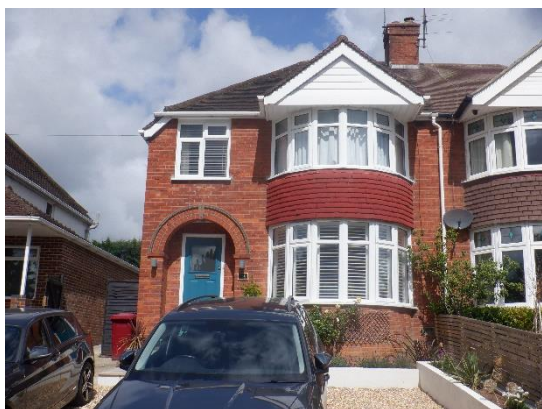
1. Front of property viewed from the south.
