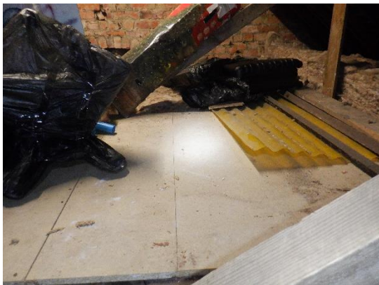
11. Part boarded floor over fibreglass insulation.
