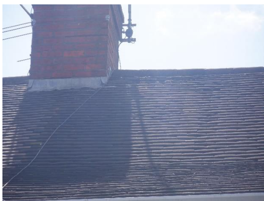
3. Concrete tiles mostly tight throughout.
