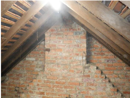
9. Roof void approx. 2 metres in height.
