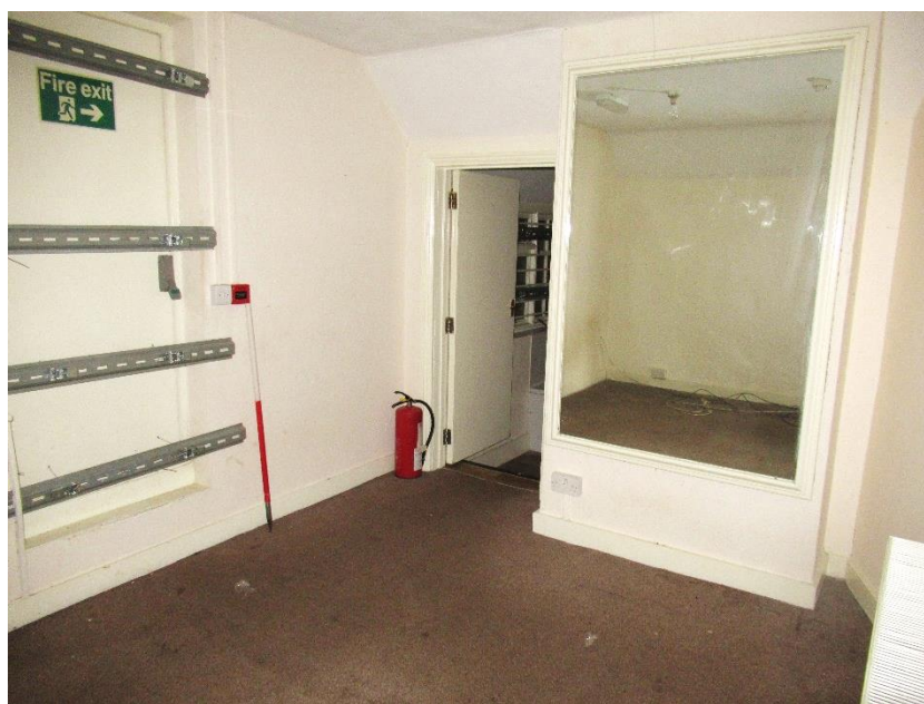
Plate 1 – First floor room of the L shape building
