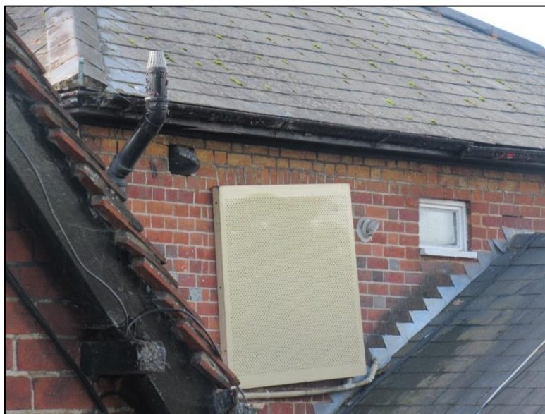
Plate E – Part north elevation showing segmental brick head to infilled window and variation in brickwork to the eaves suggesting a phase of rebuilding or alteration
