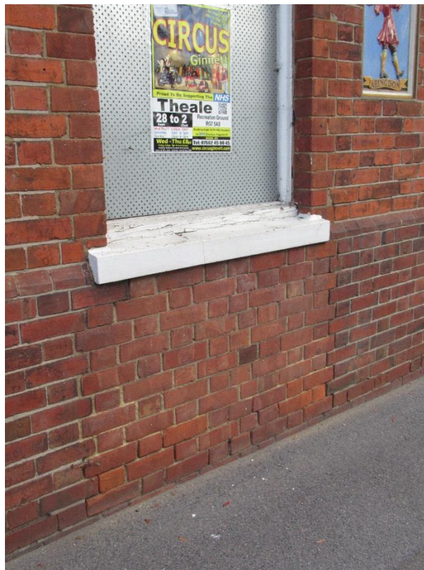
Plate 4 – Altered door opening to the centre of the south elevation of the main building
