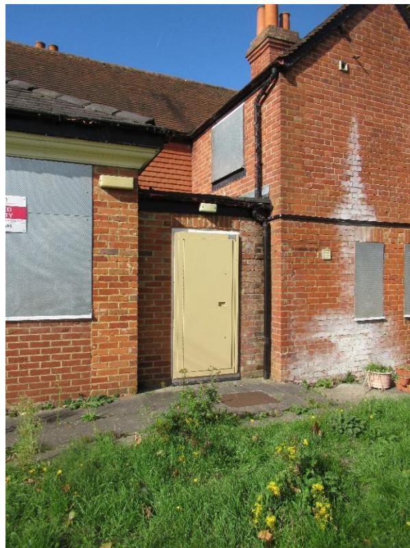
Plate 14 – Part south and west elevation of the L shape building with infill addition to the ground floor
