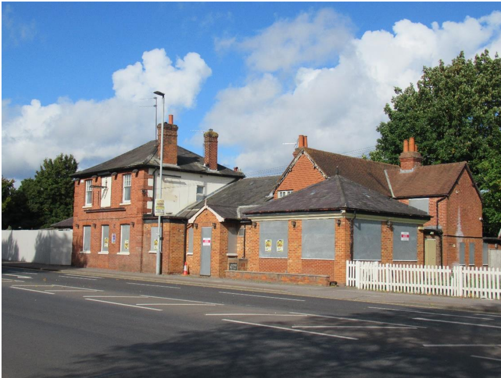
Plate 1 – South and east elevation viewed from Bath Road
