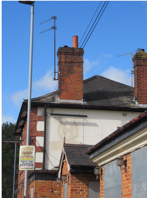
Plate 15 – First floor east elevation of the main building
