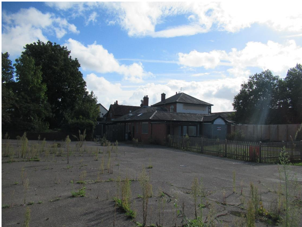
Plate 16 – General view of the west and north elevations from within the carpark area to the west
