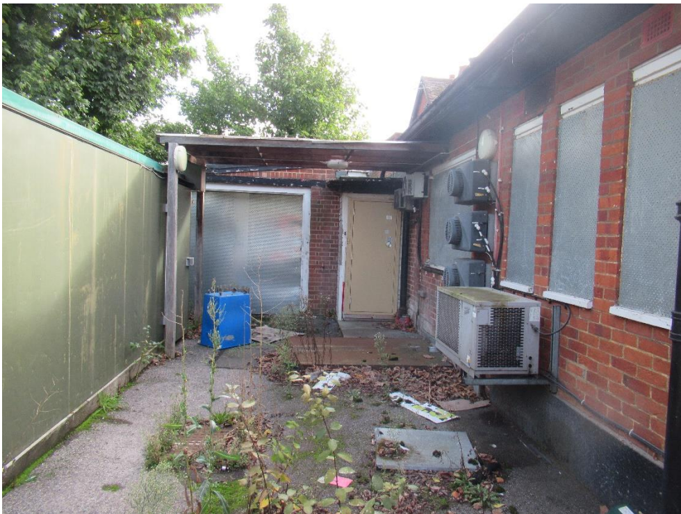
Plate 20 – Garage building and part north elevation viewed from back of house yard area
