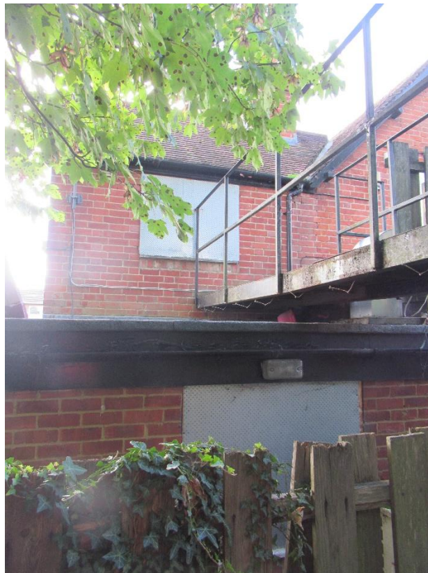
Plate 30 – Part north elevation of the L shape building
