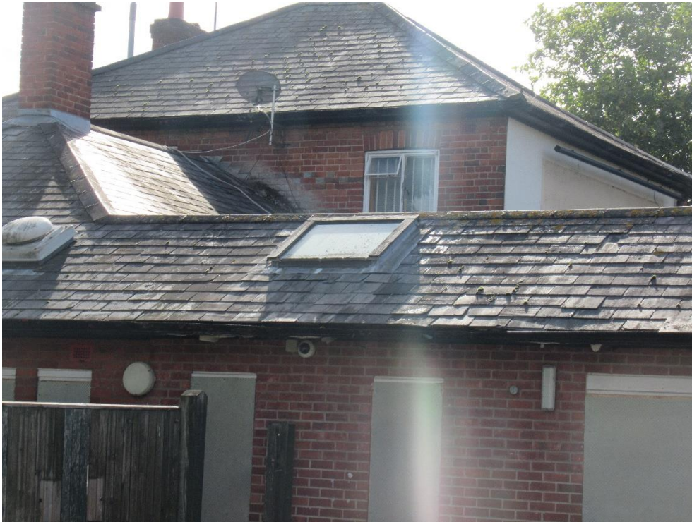
Plate 25 – Part north elevation of the main building
