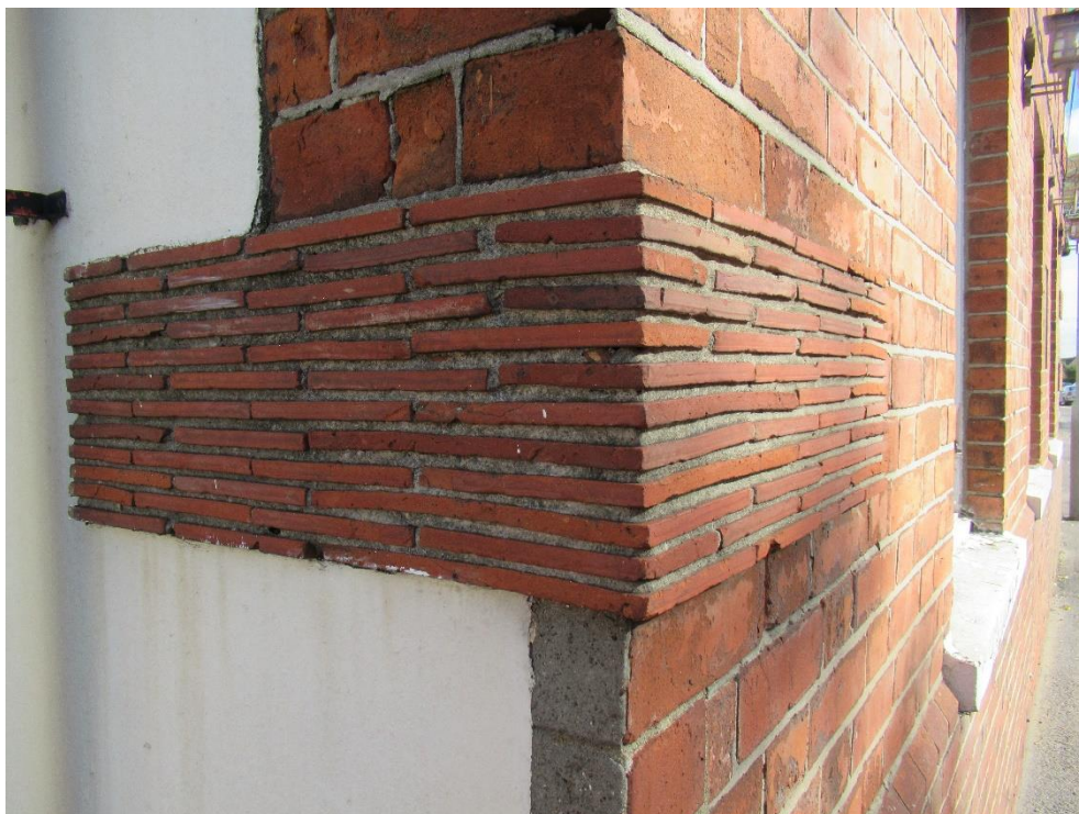
Plate 6 – Quoin detail present to the east and west corners of the south elevation of the main building
