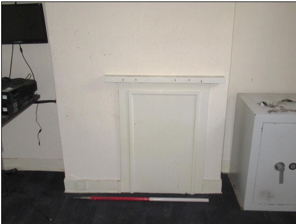
Plate H – Fireplace and chimney breast to the northwest first floor room of the main building
