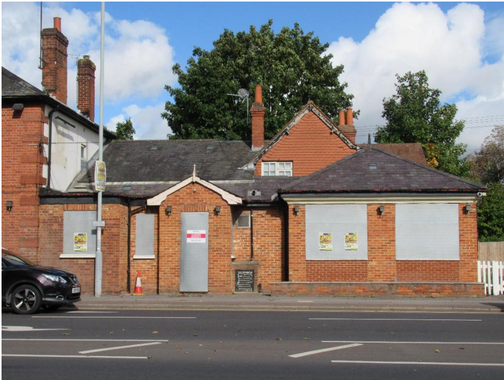
Plate 7 – Additions to the east of the main building; gabled form of the first floor of the L shape building visible to right of centre
