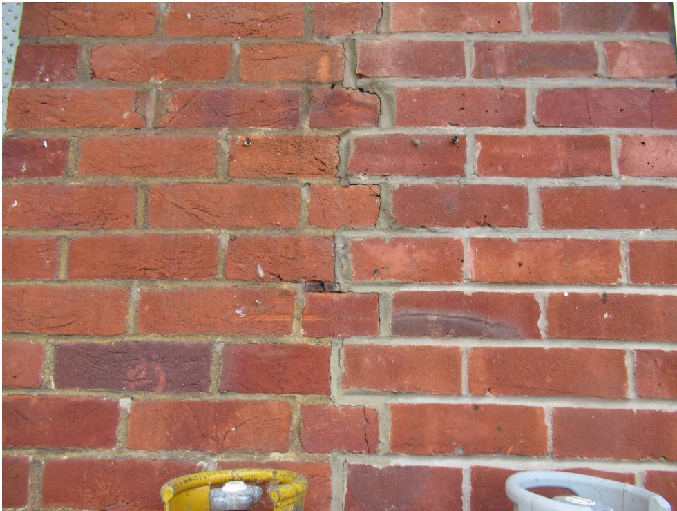
Plate 21 - Joint in brickwork visible on the north elevation between the mid-20 th century addition to the north and later 20 th century addition to the northwest corner and west
