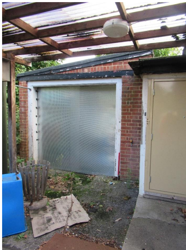
Plate 22 - West elevation of the garage addition
