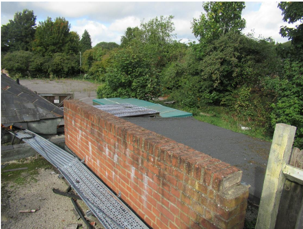
Plate 26 - Brick parapet between a later flat roof addition to the north and the flat, felt covered roof of the garage addition
