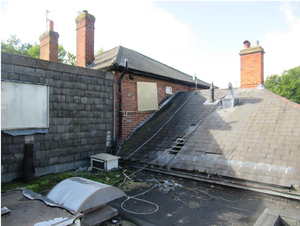
Plate 27 – Part north elevation of the main building and east roof slope of the mid-20 th century addition to the north
