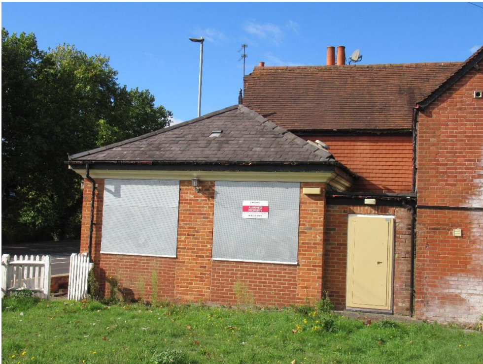
Plate 12 – East elevation of pyramidal addition
