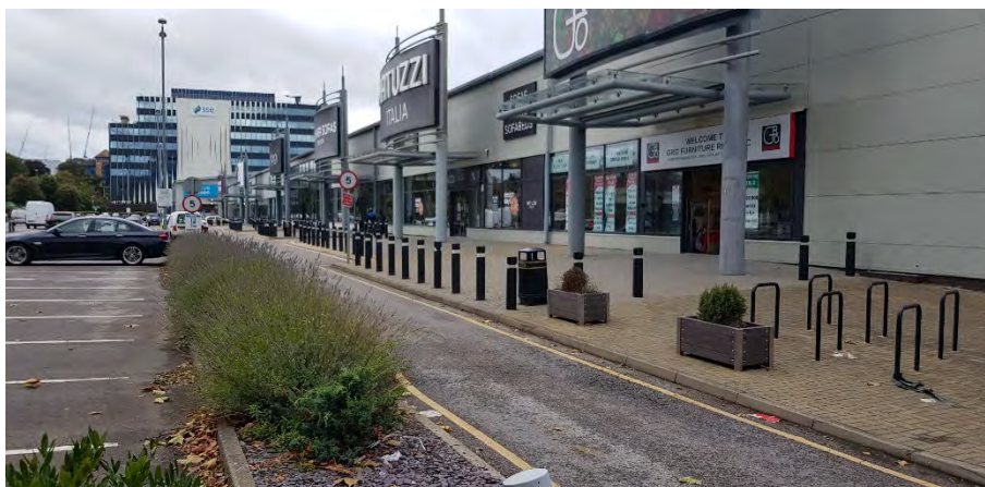
Photograph 9: Hardstanding, introduced shrub and building were the predominant habitats on Site
