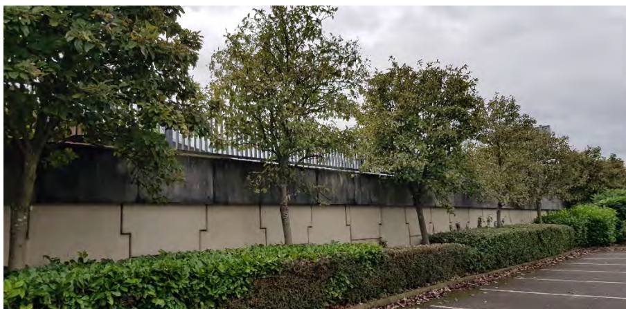
Photograph 12: Scattered trees and shrubs along southern boundary wall.
