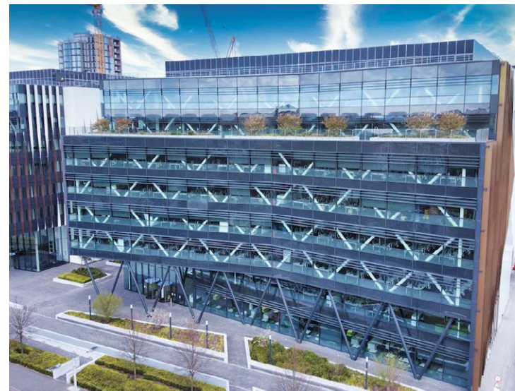
Offices at Forbury Place (1-3 Forbury Place, Reading, RG1 3)
