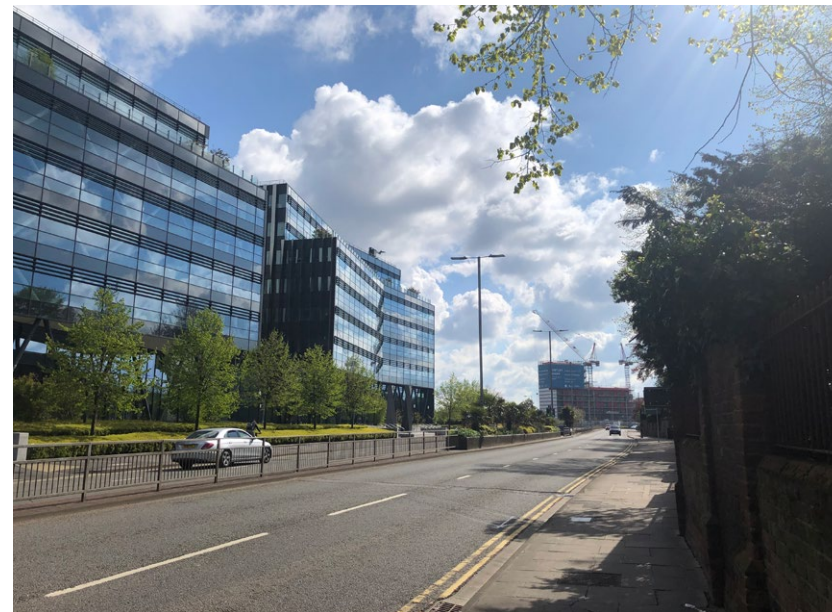
View along Forbury Road towards the east and the site
