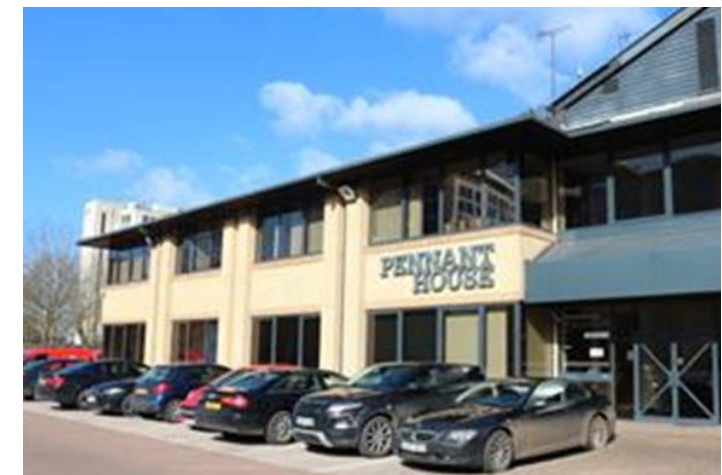
Napier Court Offices (Pennant, Hawker and Emerald House, Reading, RG1 8)
