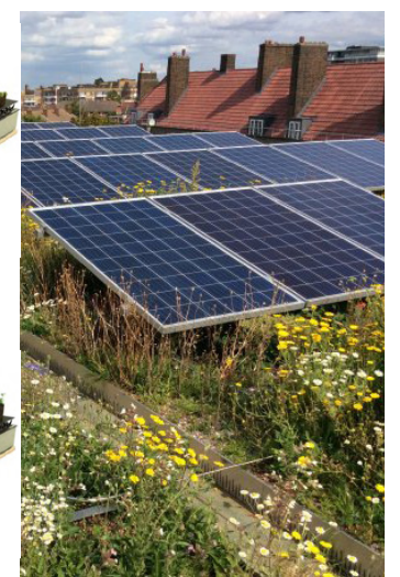
Typical rooftop combining PV & biodiverse planting
