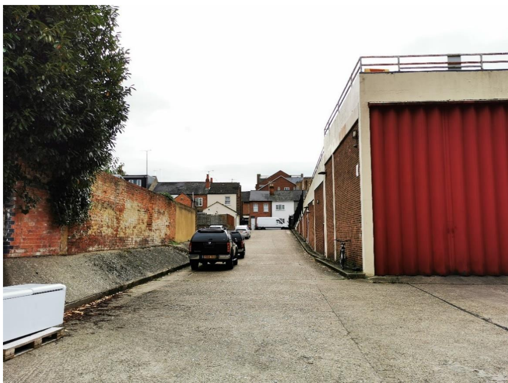
Plate 2: External view looking south from the lower carpark towards the east elevation wall and north elevation warehouse door.
