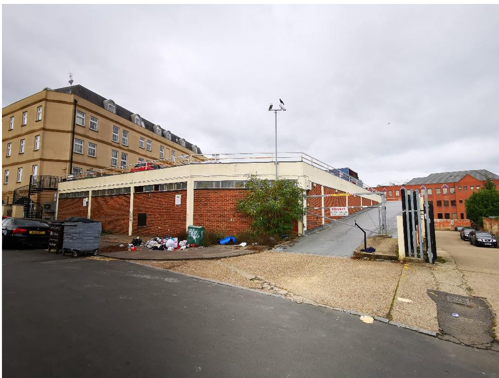
Plate 1: External view looking northwest from Upper Crown Street towards the north elevation.
