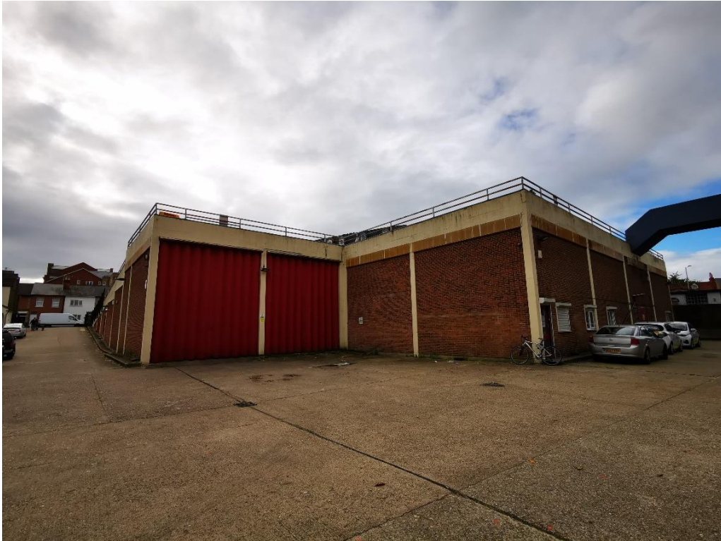
Plate 3: External view looking southwest towards the north elevation from the lower carpark.
