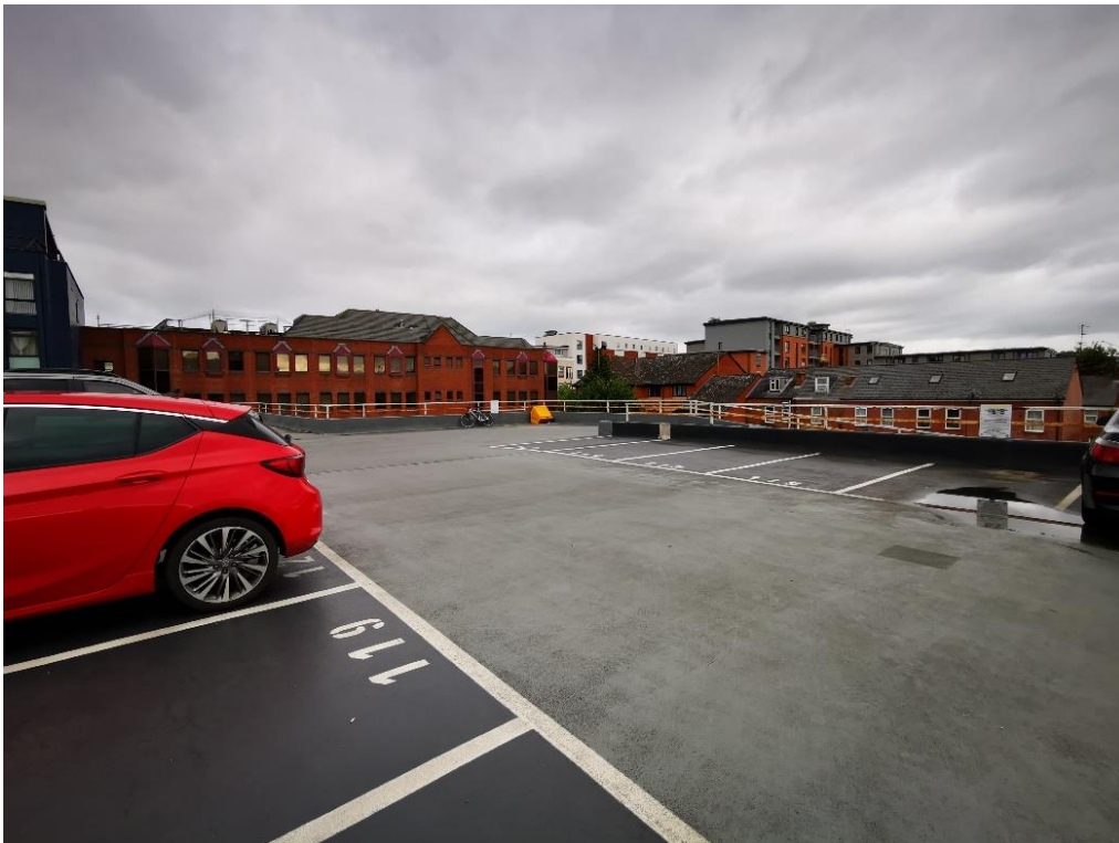
Plat 4: External view looking northeast from the rooftop carpark.
