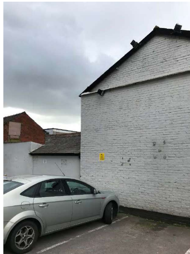
Plate 18: East elevation of Area 1a.
