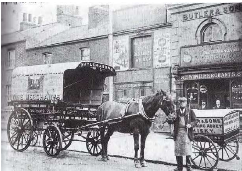
Plate 14: Photograph of the east end of the building c.1900.
