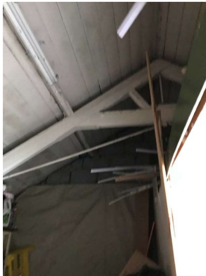
Plate 33: Roof structure within Building 2.
