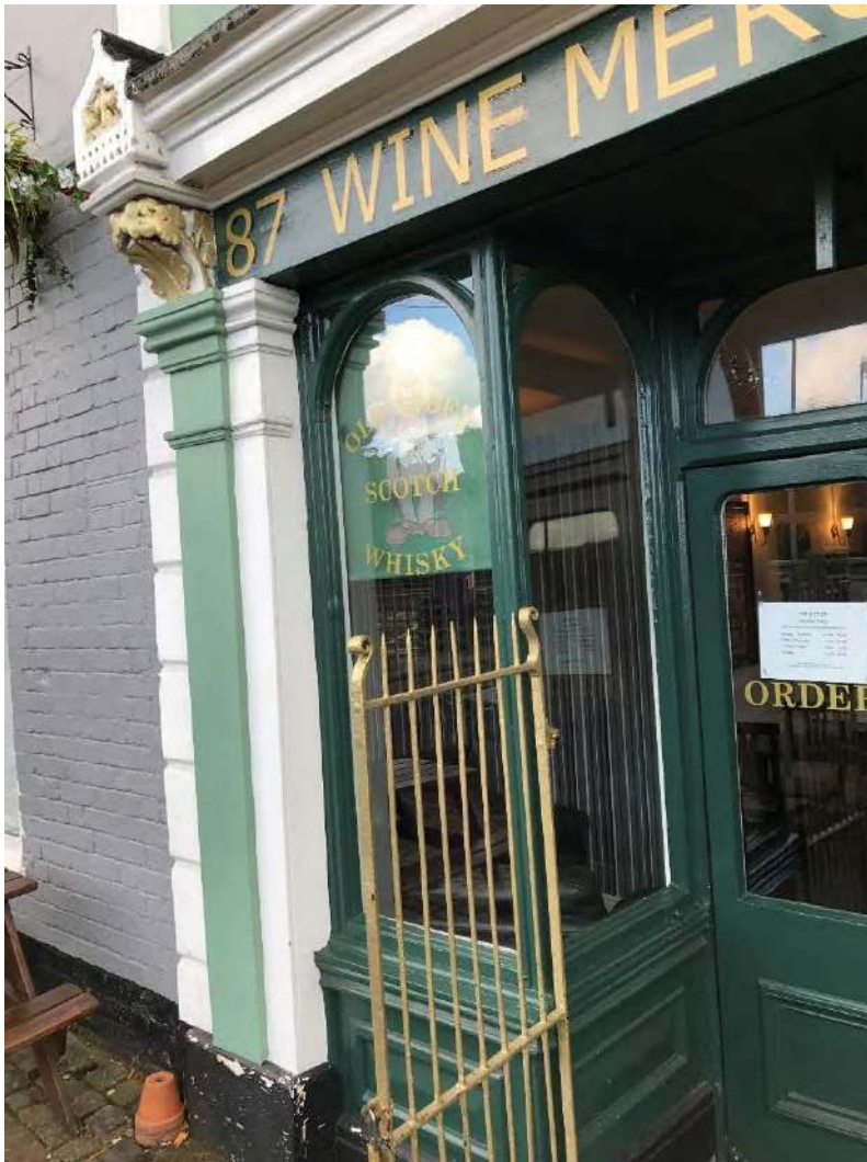
Plate 24: Detail of the shop frontage of Area 1b.
