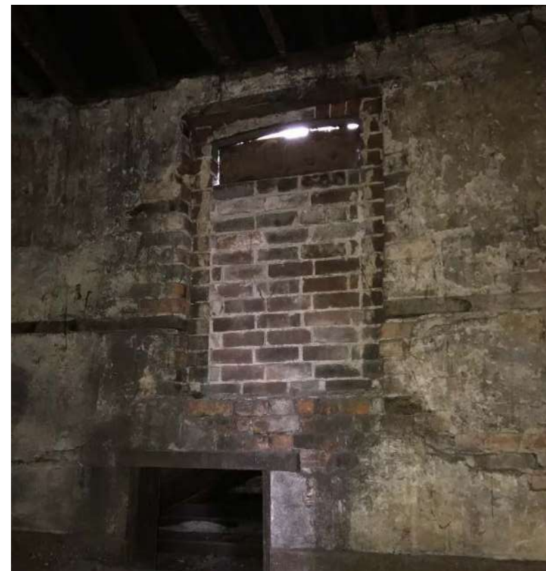
Plate 22: Blocked in opening on the south elevation of the first floor of Area 1a.
