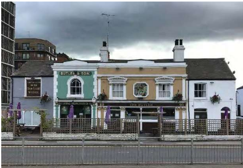
Plate 16: Principal, north, elevation of the main public house building.
