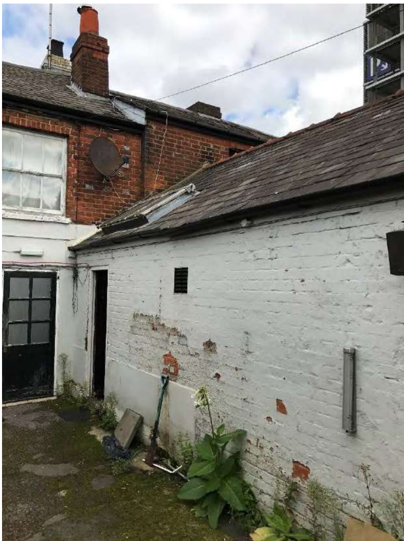
Plate 32: West elevation of Building 2.
