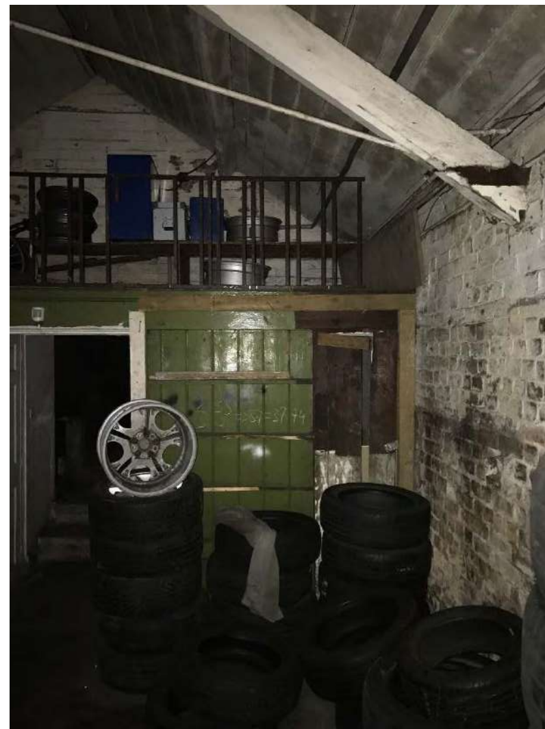
Plate 35: View north within the southern end of Building 2.
