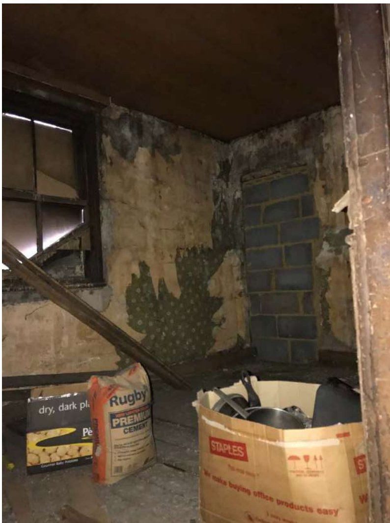
Plate 26: Blocked in former opening between Areas 1b and 1c on the first floor of Area 1b, and window on the southern elevation.
