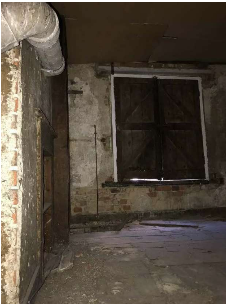
Plate 23: Blocked in opening on the north elevation of the first floor of Area 1a.
