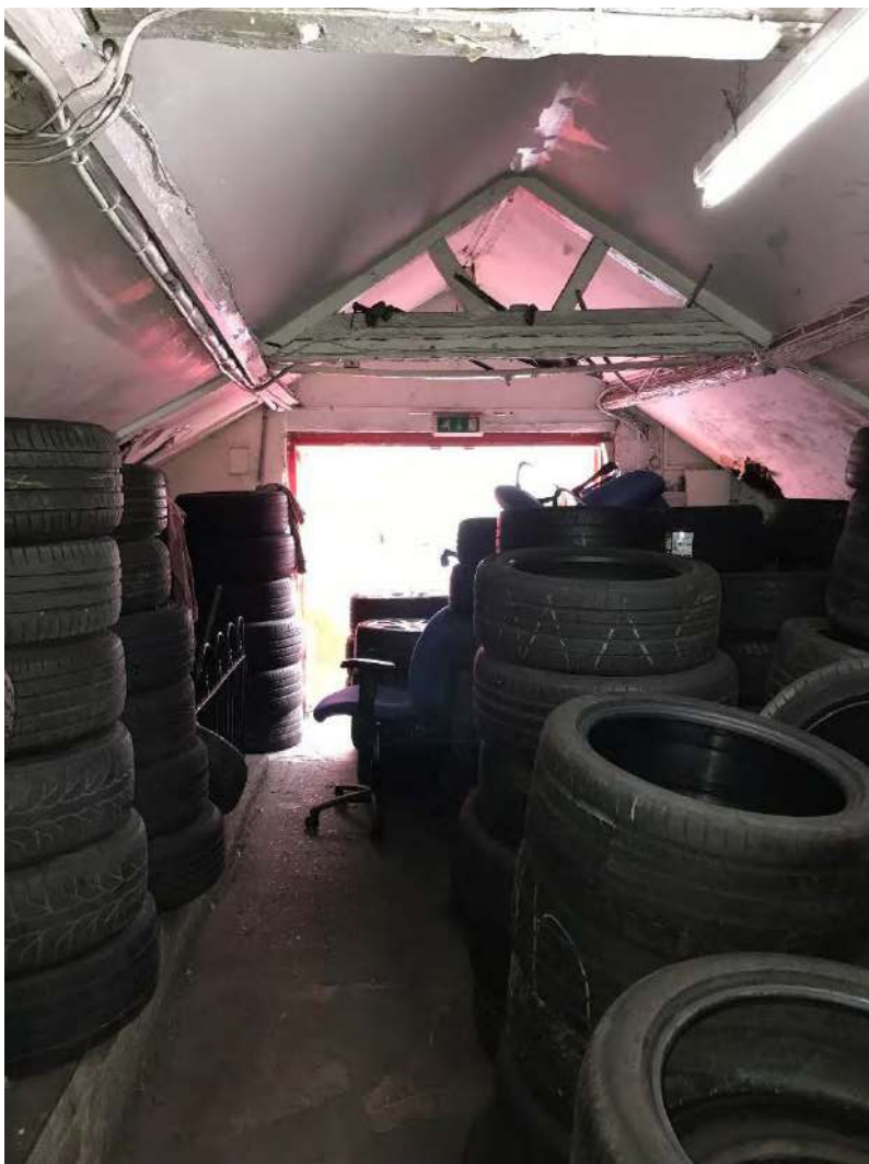
Plate 42: View east within Building 4.
