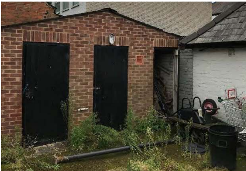
Plate 46: North elevation of Building 7.
