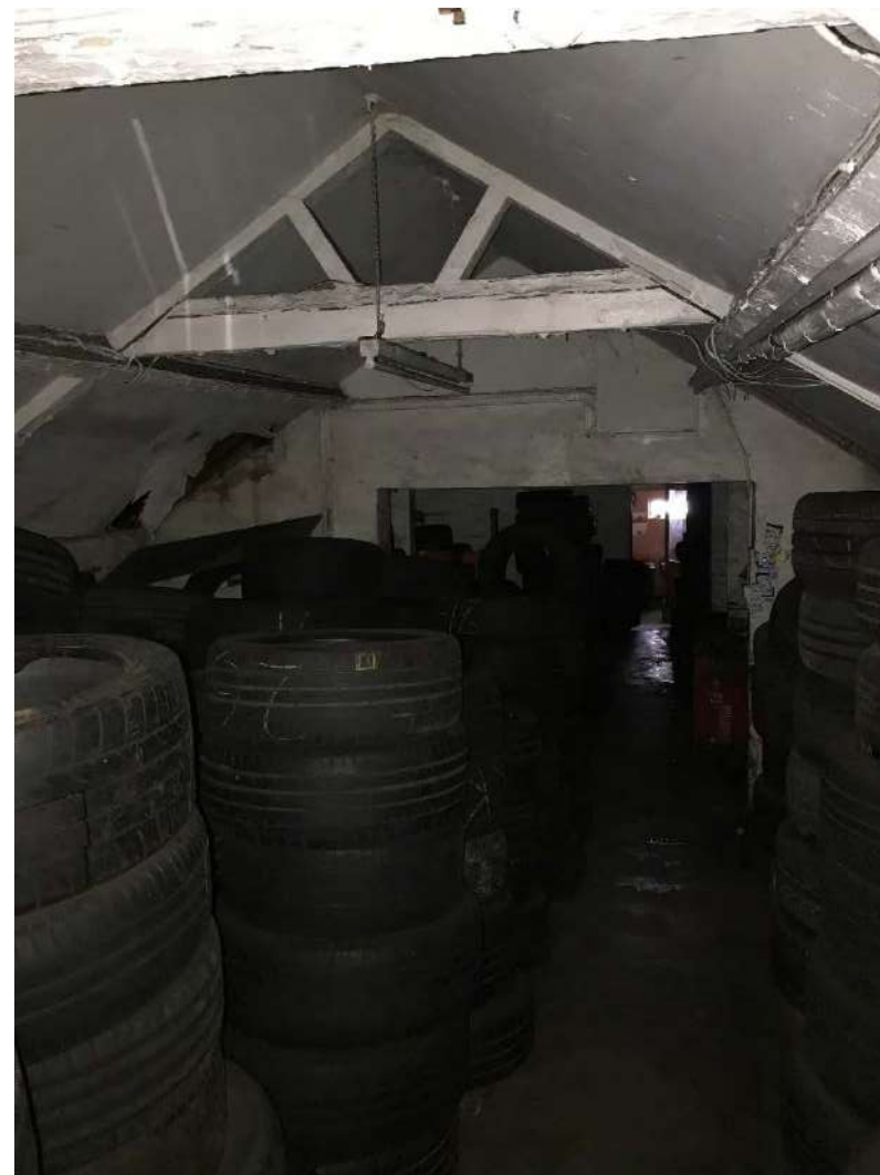
Plate 43: View west through Buildings 4, 5 and 6.
