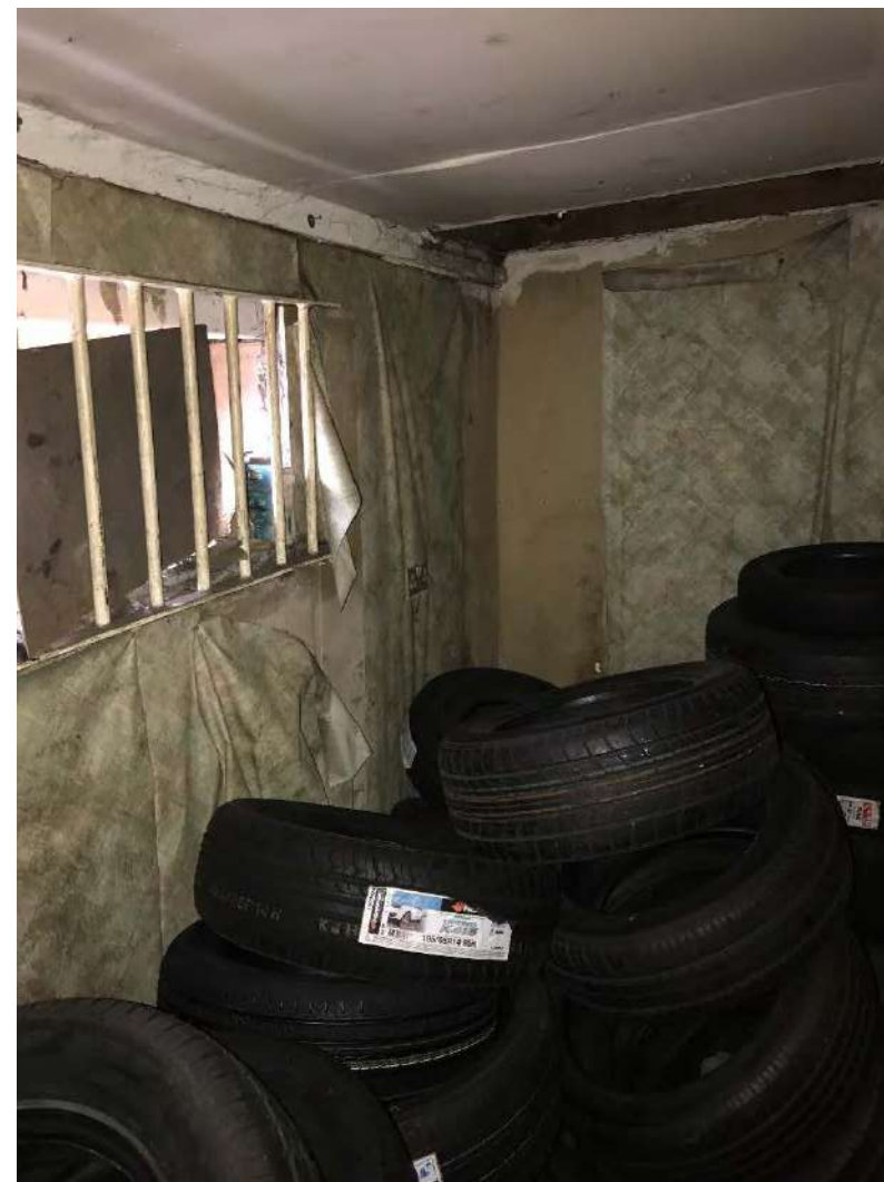
Plate 47: Interior of Building 8 facing northwest.
