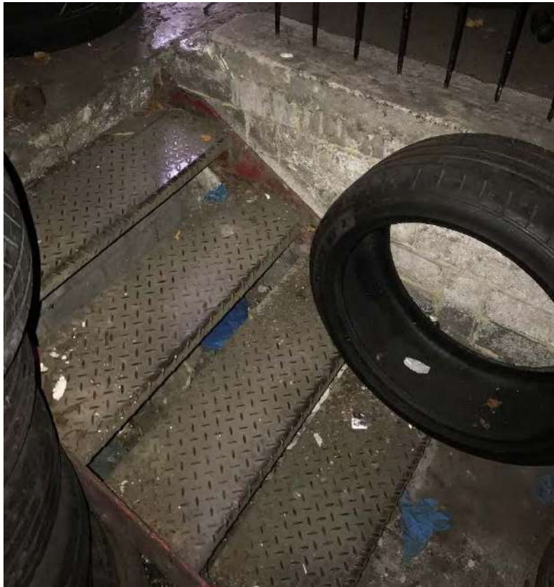
Plate 36: Steps providing access between Buildings 3 and 4.
