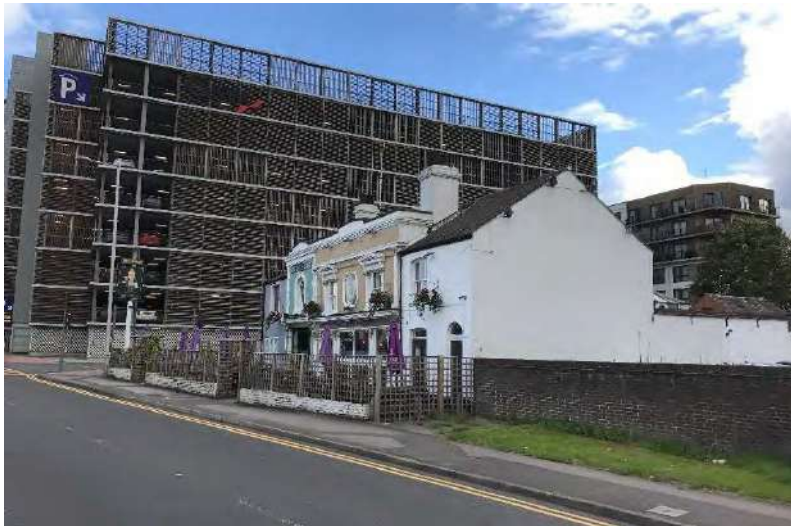
Plate 2: The Site as seen from the northwest.
