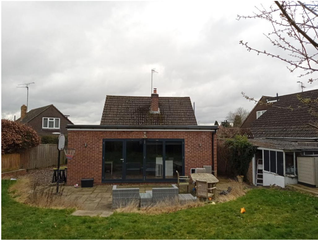
Figure 2: Existing Rear Elevation with single storey rear extension (site visit 27 February 2023)
