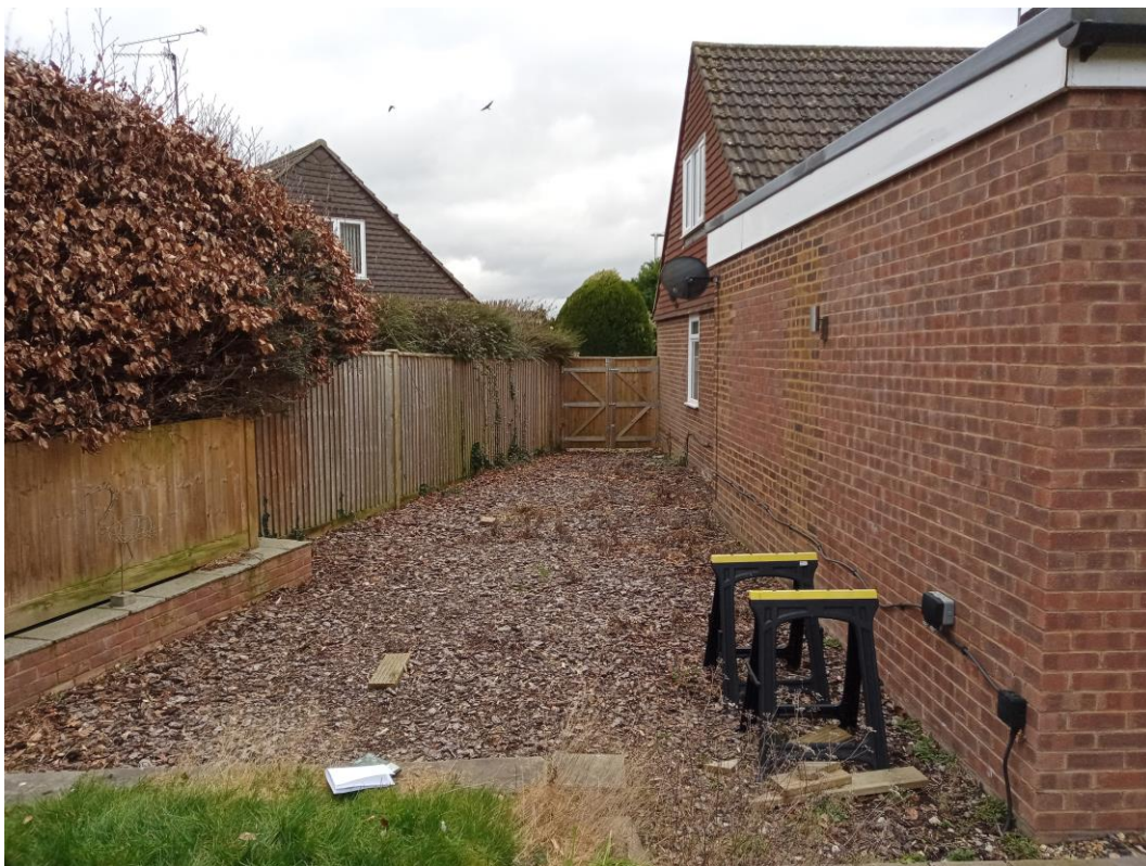
Figure 3: Eastern side elevation (site visit 27 February 2023)
