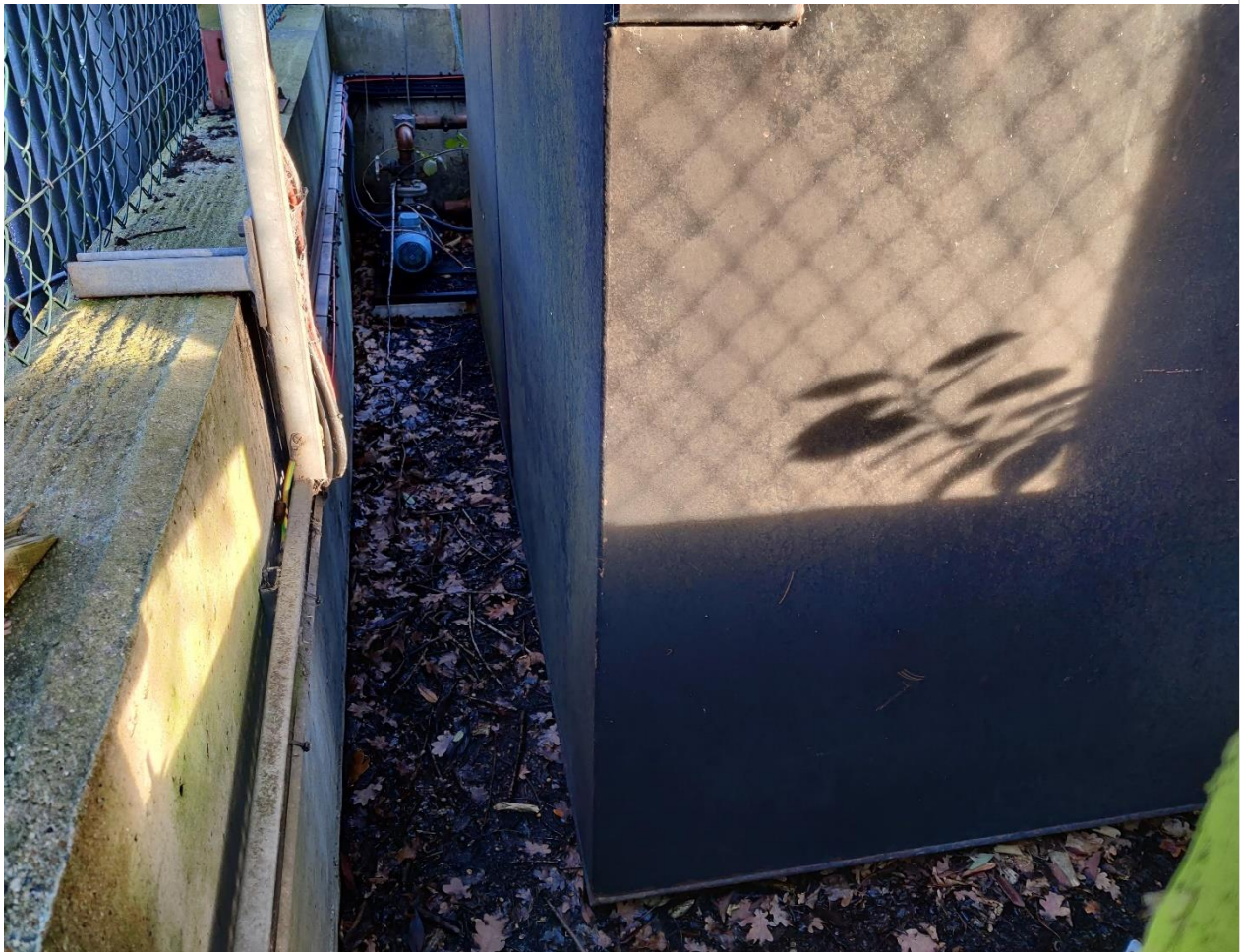
Plate 4 - Inside AST cage, pump noted at rear of the cage and no evidence of spillages.
