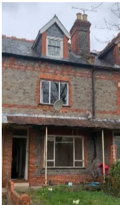
Site visit photo: front elevation
