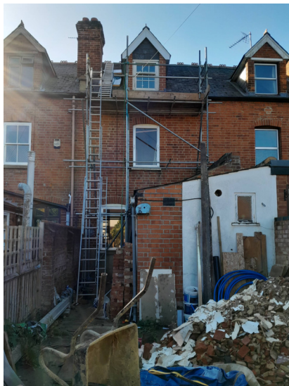
Site visit photo: rear elevation
