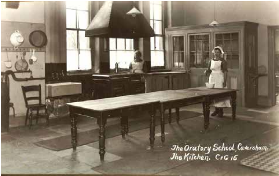
Figure A1.79 1930s Oratory School archive kitchen
