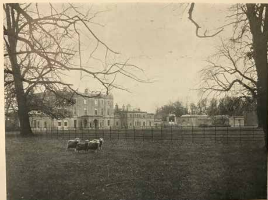
CAVERSHAM PARK.—THE ENTRANCE FRONT.
