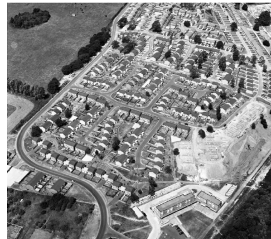
Figure A1.94 1970 aerial photo
