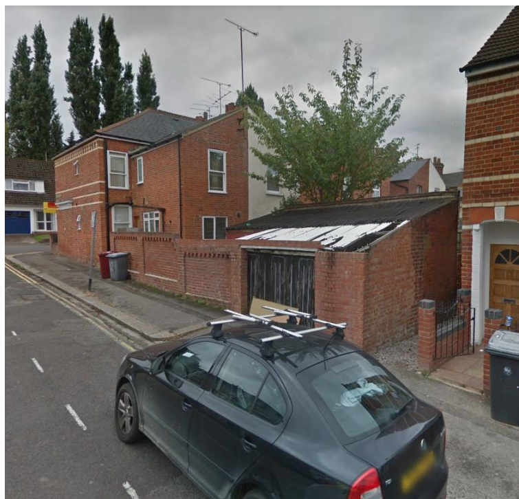
The existing outbuilding at the rear of 2 Gloucester Road, as seen from Elm Park Road. Image taken from Google Maps on 22.08.2023.
