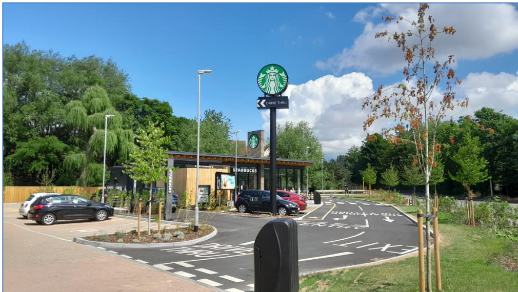
Fig 1. Site photo taken by case officer on 21/06/2023.
