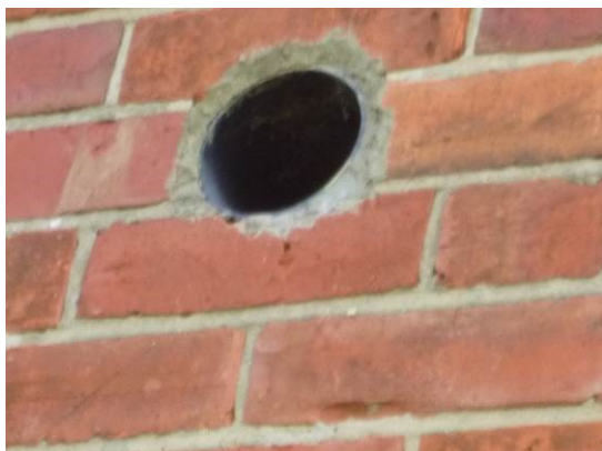
7. Hole with pipe insert in gable wall (west elevation).
