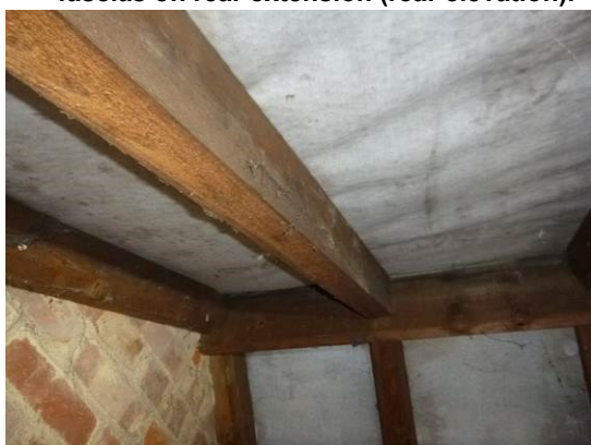
11. Breathable roofing membrane and lightly cobwebbed ridge (roof void).
