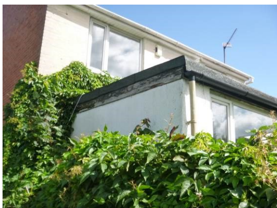
9. Bituminous flat roof and flush timber fascias on rear extension (rear elevation).
