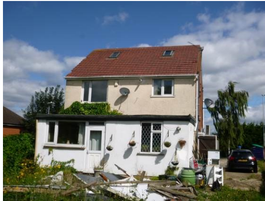
2. Rear of property viewed from south.
