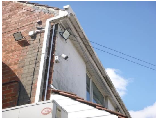
6. Intact and tight uPVC soffits (front elevation).
