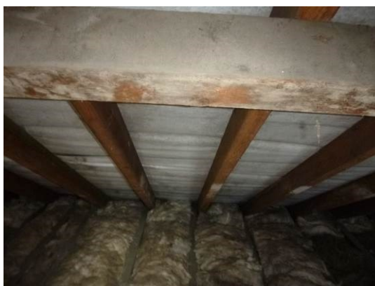
12. Eaves filled with fibreglass insulation (roof void).
