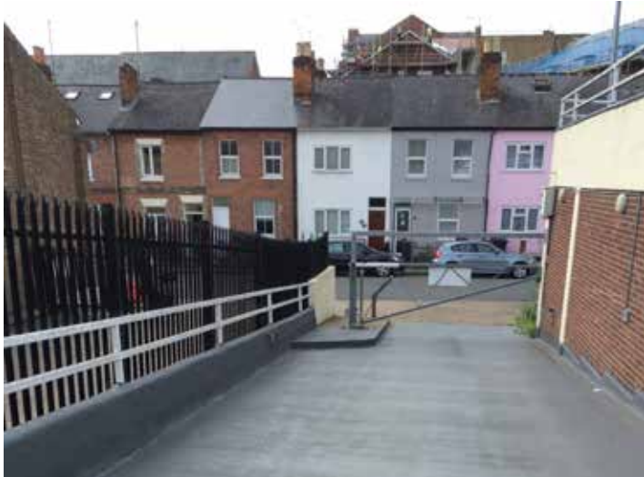
Vehicle ramp to car park deck
