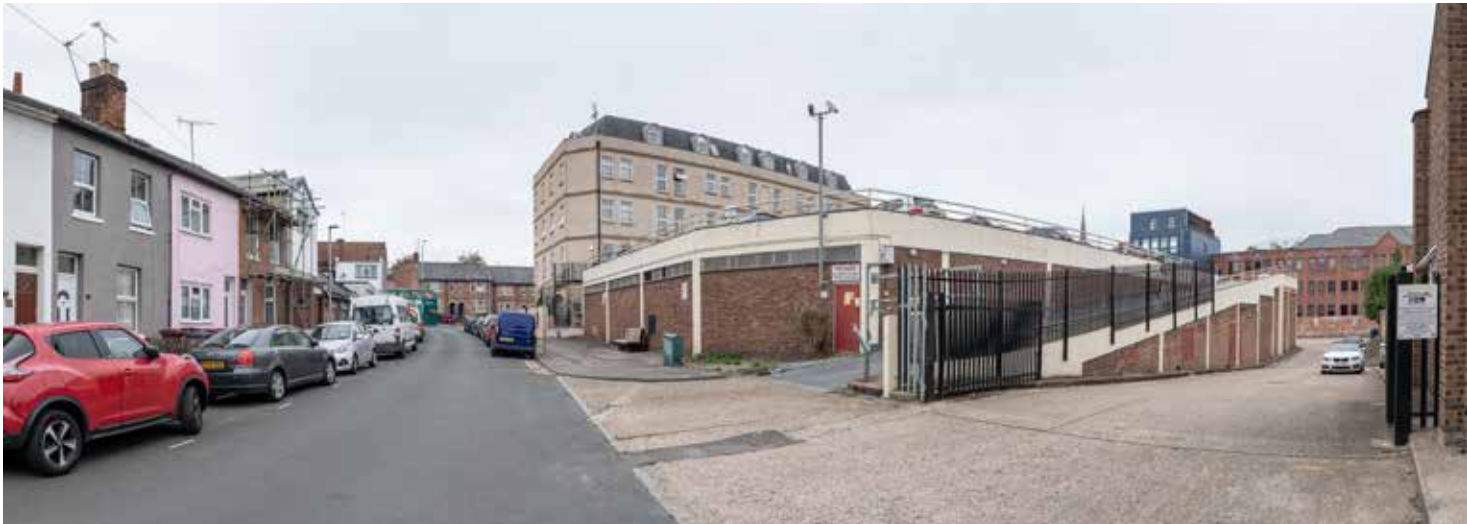
Upper Crown Street frontage
