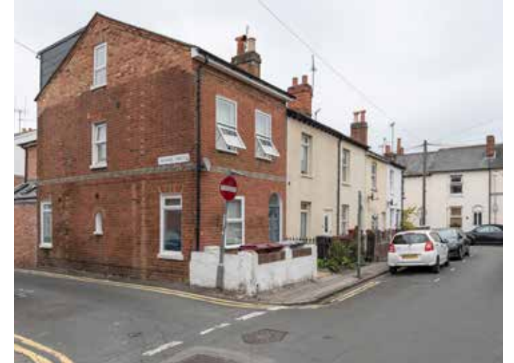
Upper Crown Street
