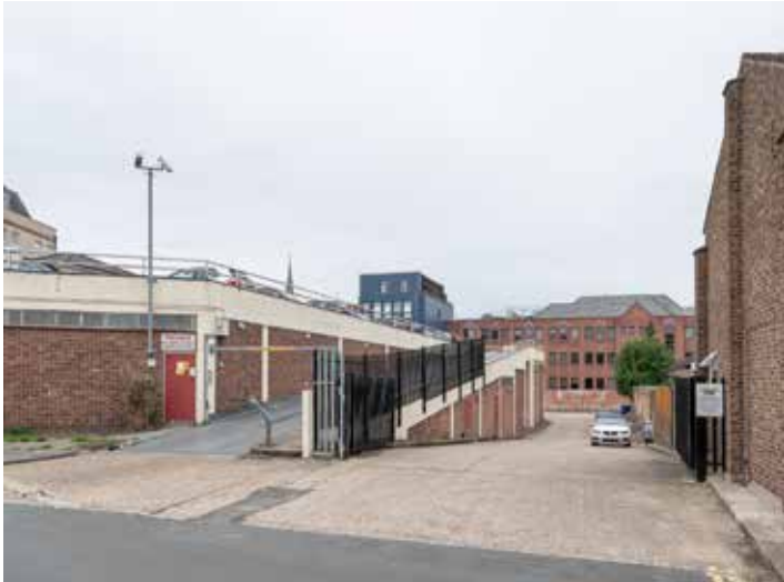
Existing ramped entrance
