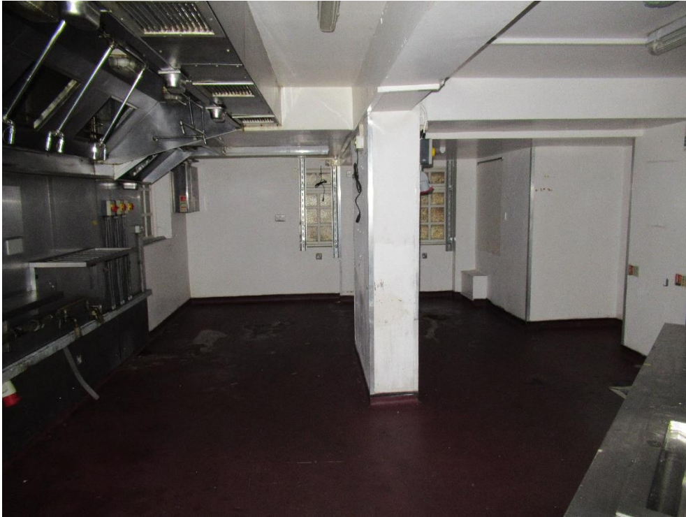
Plate 103 – View east through the ground floor of the kitchen
