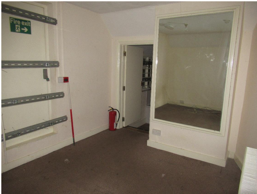
Plate 93 - Interior of the north first floor room of the L shape building looking northeast
