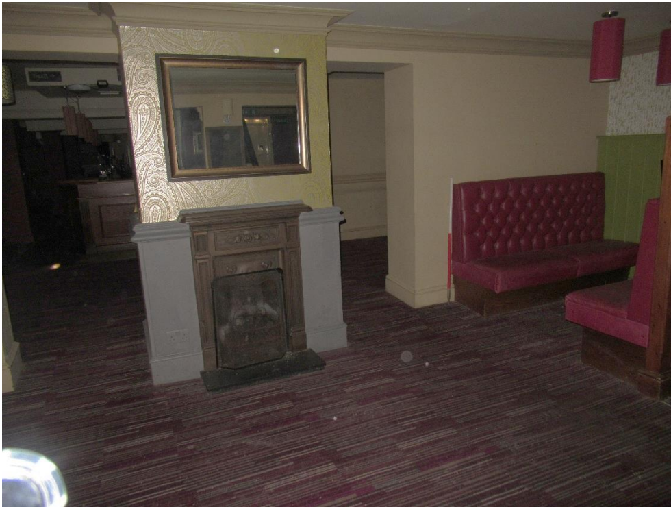
Plate 41 – Interior view of the ground floor of the L shape building with section of original west elevation retained to the right of the image
