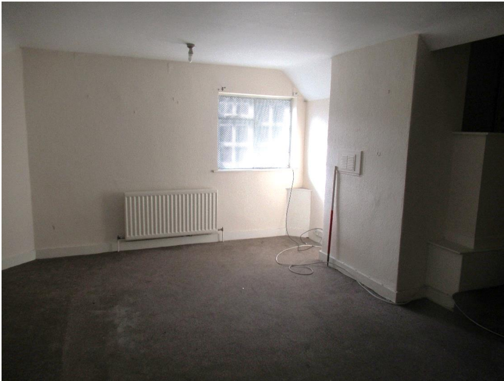
Plate 89 – Interior of the south first floor room of the L shape building looking southwest with chimney breast to the right of the image
