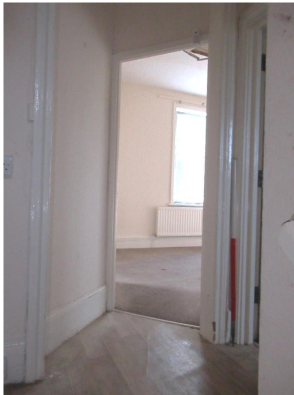
Plate 70 – First floor landing area of the main building with splayed entrance to the south rooms
