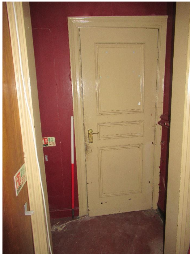
Plate 58 – Timber panel door to the cellar area
