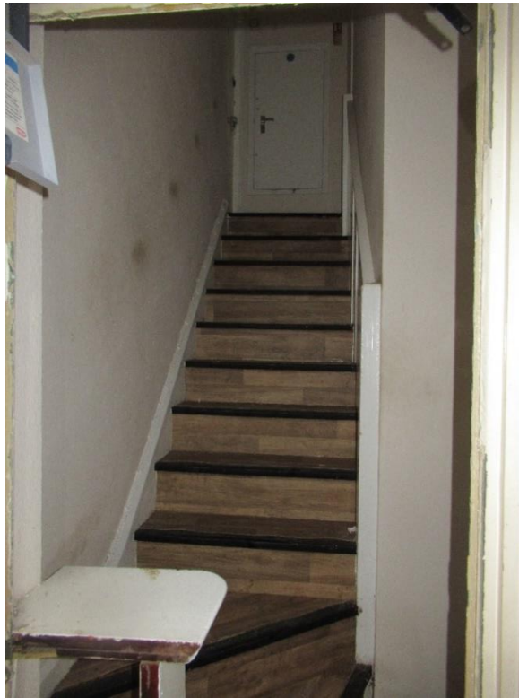
Plate 69 – Staircase to the first floor
