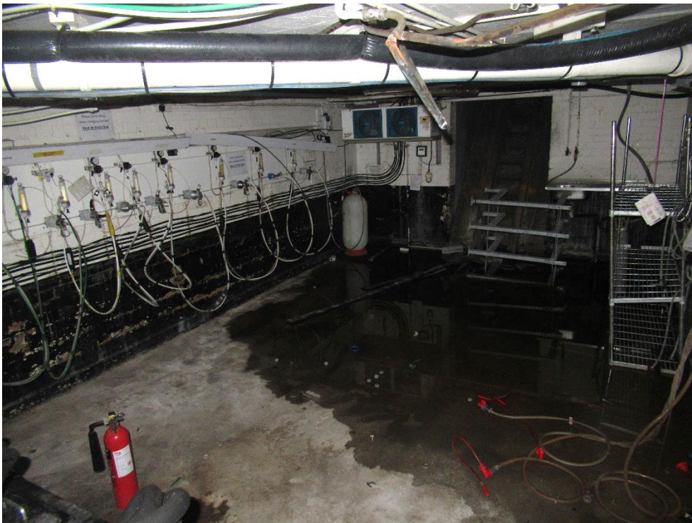
Plate 60 – Cellar area located below part of the ground floor of the mid-20 th century addition to the north
