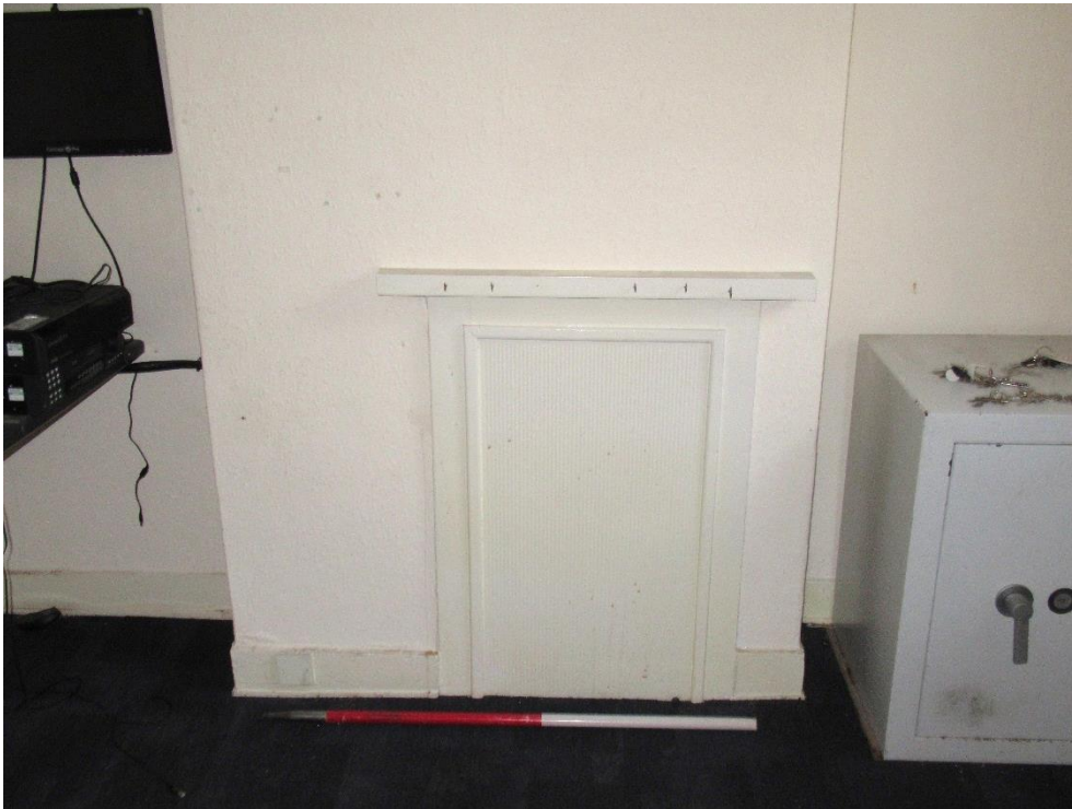
Plate 83 – Fire surround to the west floor of the northwest first floor room of the main building
