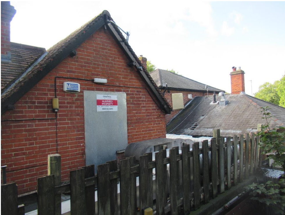
Plate 32 – Door opening inserted to the north elevation of the L shape building
