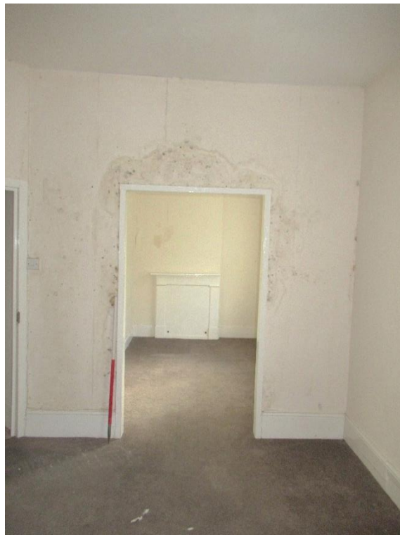
Plate 74 – Later opening inserted within original partition wall between the southwest and southeast first floor rooms of the main building
