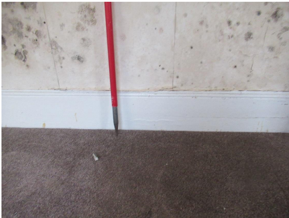
Plate 76 – Skirting board detail to the southwest first floor room of the main building
