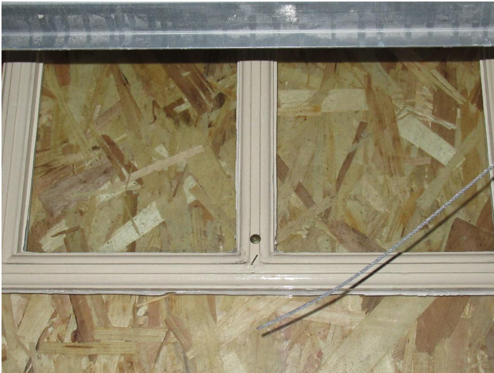
Plate 49 – Ovolo moulded glazing bars typical to the ground floor windows of the south elevation of the main building
