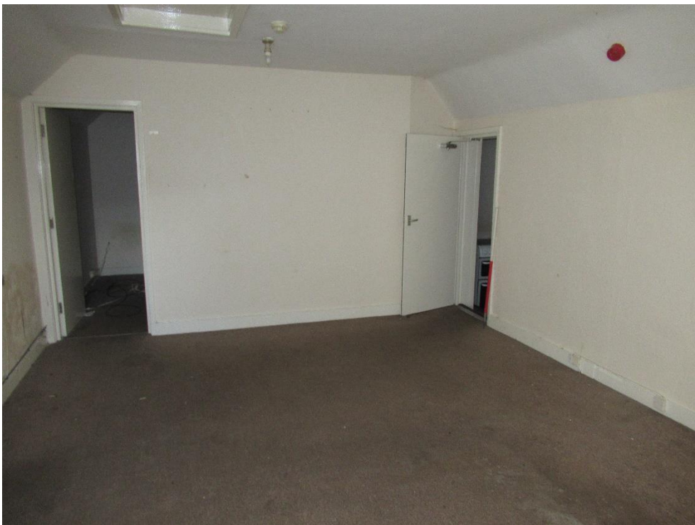
Plate 90 - Interior of the south first floor room of the L shape building looking northeast
