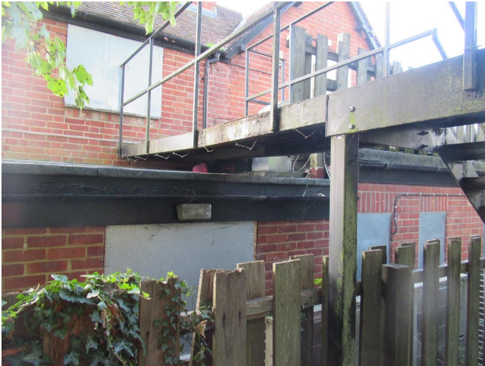
Plate 31 – Part north elevation of the L shape building
