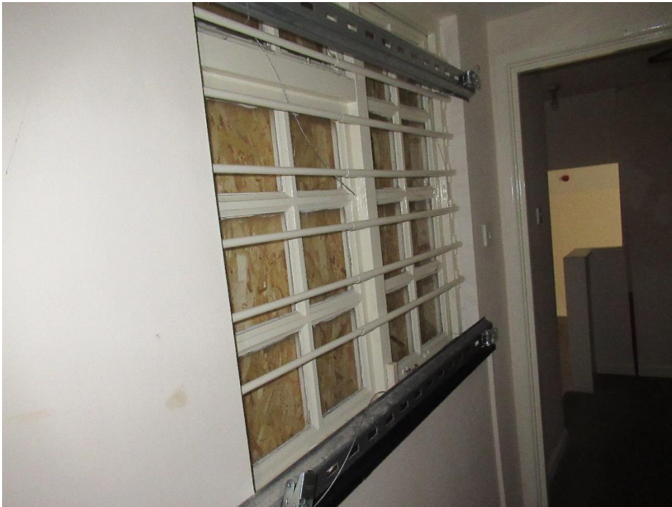
Plate 87 – Interior view of later first floor window within the north elevation of the two-storey addition to the west
