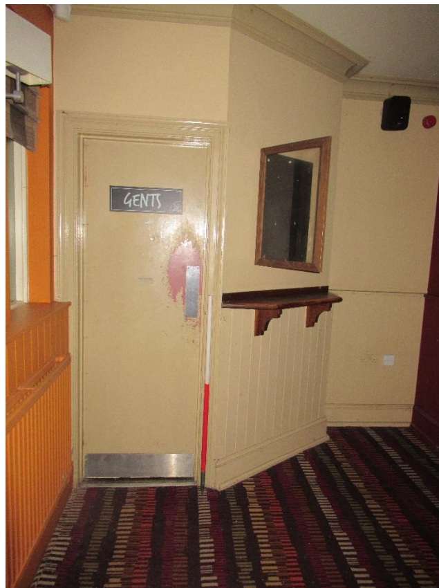
Plate 56 - Door opening to the male WCs located within the mid-20 th century addition to the north of the main building
