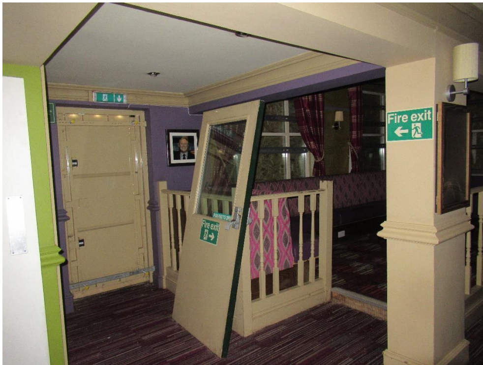
Plate 43 – View from within the ground floor of the L shape building into a later addition to the west
