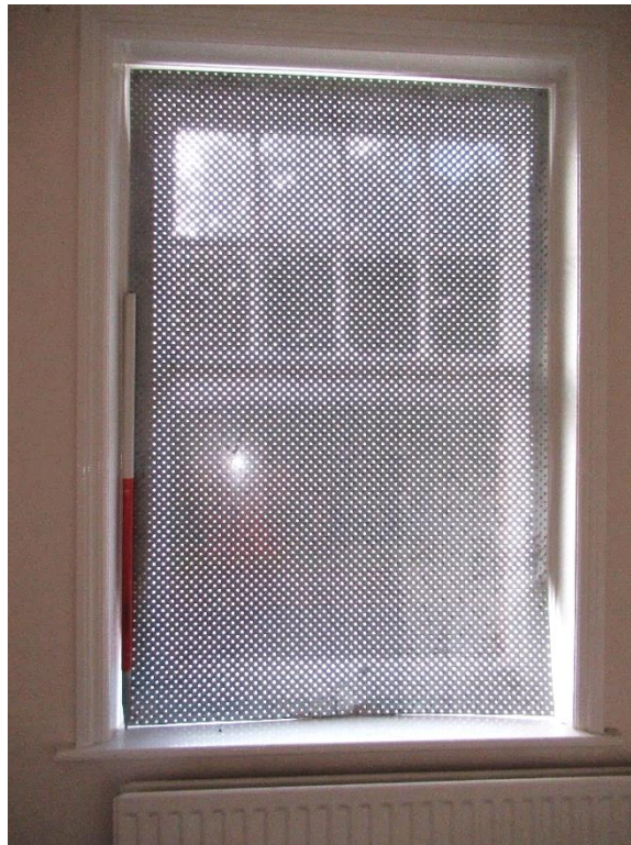
Plate 81 – Interior view of the eastern first floor window to the south elevation
