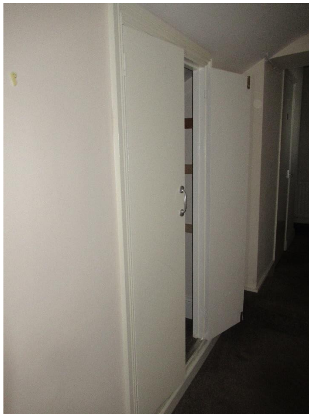
Plate 88 – Cupboards located to the south of the first-floor access corridor between the main building and the L shape building
