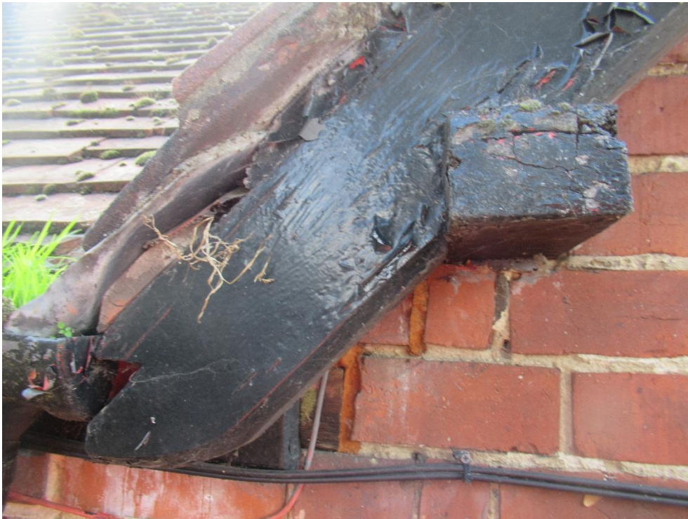
Plate 33 – Timber purlin foot and bargeboard detail to the verges of the north elevation of the L shape building
