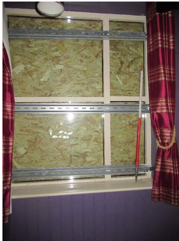
Plate 47 – Interior window detail to the windows within the pyramidal addition to the east
