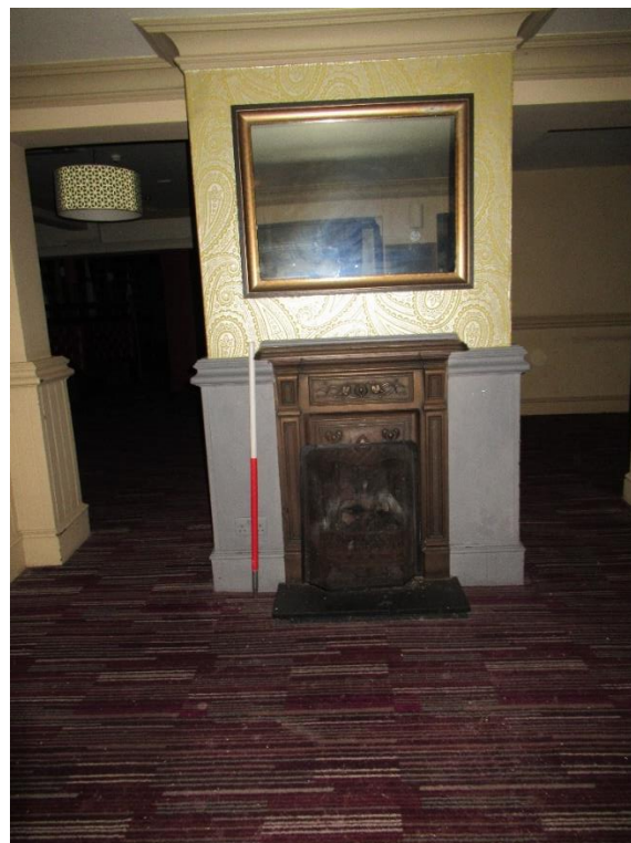
Plate 40 – Renewed fireplace within original location with chimney breast to the west elevation of the L shape building
