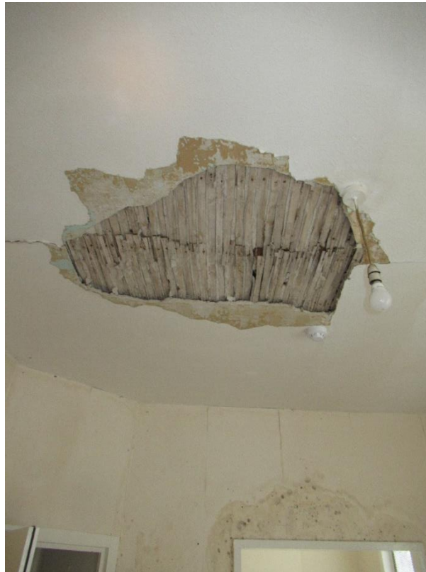
Plate 77 – Original lath and plasterwork to the first-floor ceiling of the main building
