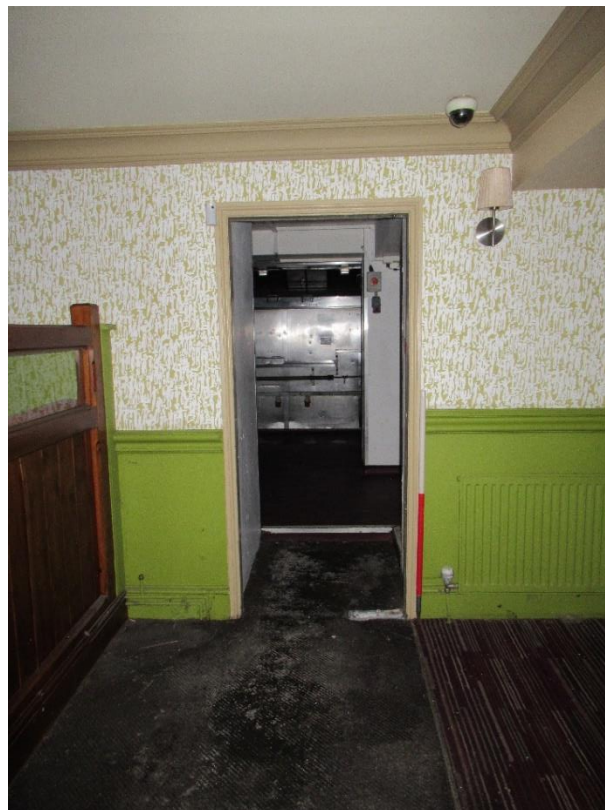
Plate 42 – Door opening (to kitchen) within a modern partition inserted to the ground floor of the L shape building
