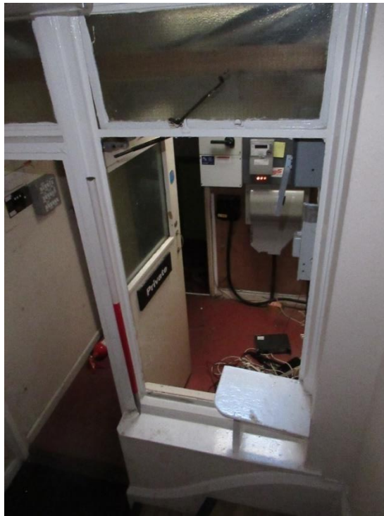
Plate 65 – Remains of glazed screen frame between the office and the staircase
