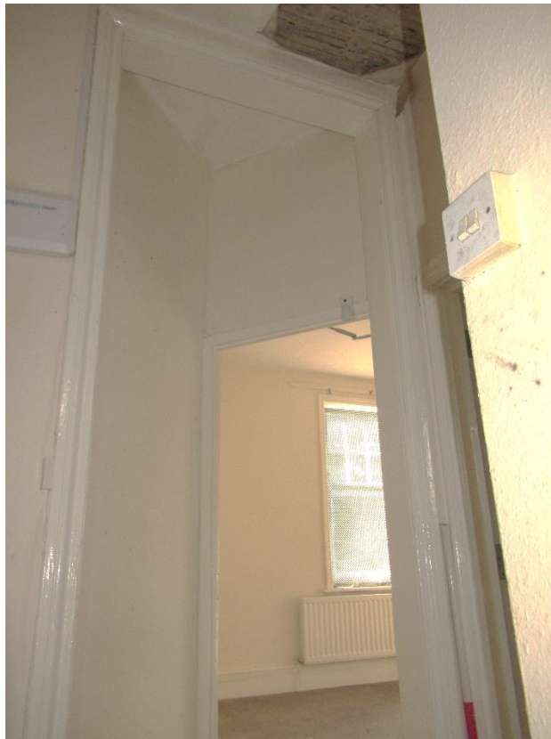
Plate 71 – Surround detail to the opening to the south rooms from the first-floor landing of the main building
