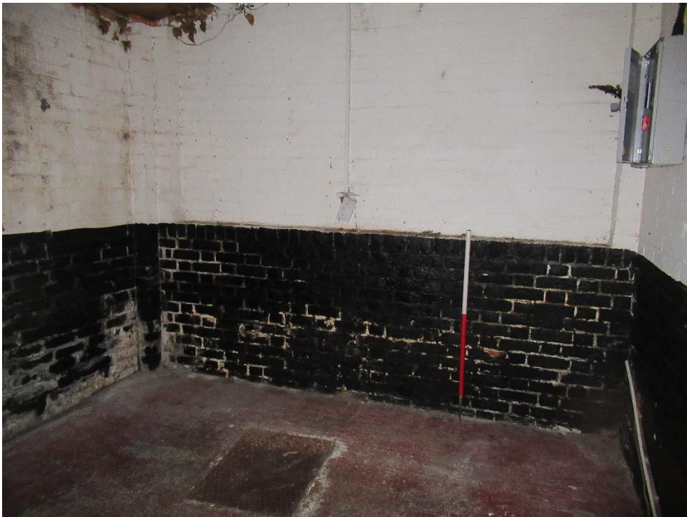
Plate 100 – Interior view of the original garage addition
