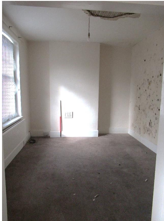
Plate 73 – First floor room to the southwest of the main building with off centre chimney breast
