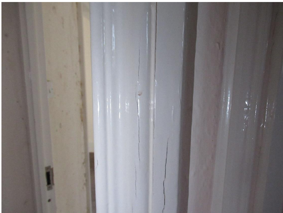
Plate 72 – Architrave detail to the surround to the opening to the south rooms
