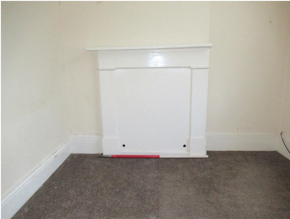
Plate 79– Fire surround to the east wall of the southeast first floor room of the main building
