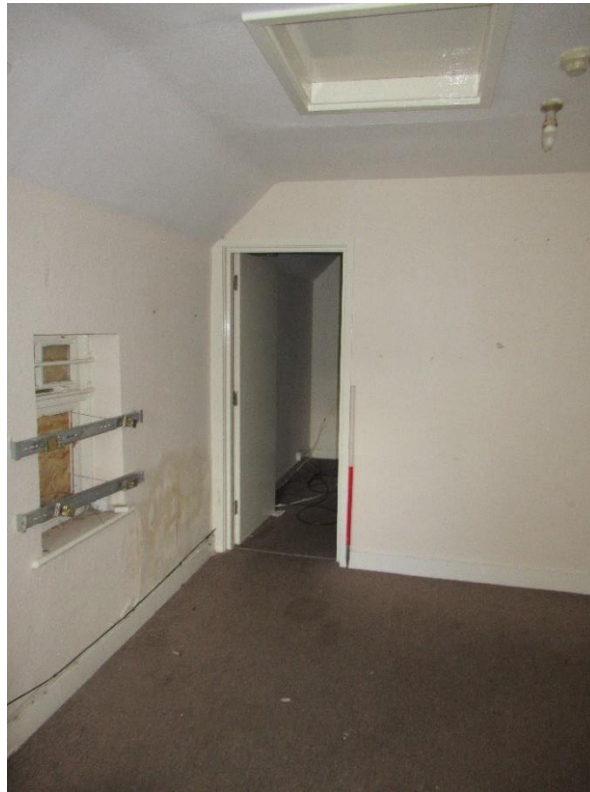
Plate 91 - Interior of the south first floor room of the L shape building looking north
