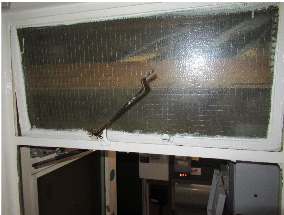
Plate 64 – Metal framed top light window to the glazed screen between the office and staircase
