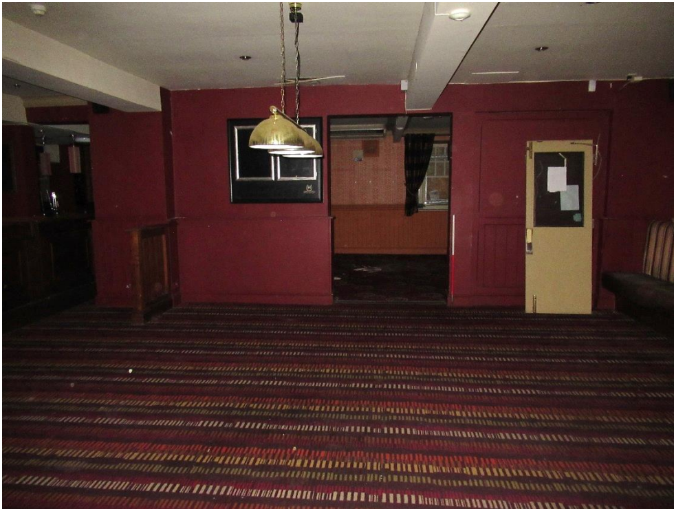
Plate 53 – View south through the ground floor of the west addition
