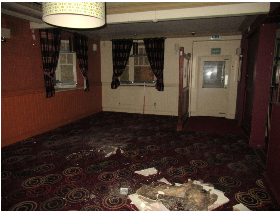
Plate 52 – Interior of the west addition
