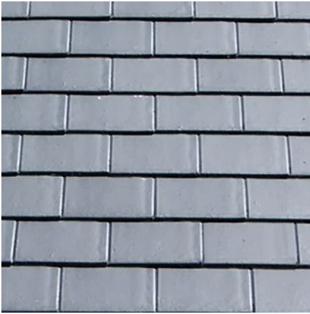
01) GREY ROOF TILES TO NEW ROOF
