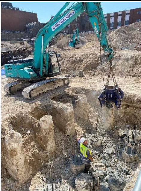
Photo 5 – Breaking out of pile caps within the concrete core base in the central west of the site.
