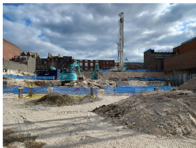
Photo 9 – View facing south across the site. Stockpiles of concrete obstructions observed in the central south of the site.
