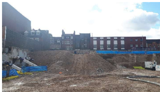
Photo 2 – Ramp material in centre east of the site which will eventually be disposed of off-site.
