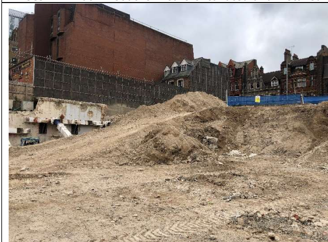
Photo 3 – Ramp material in centre east of the site which will eventually be disposed of off-site.
