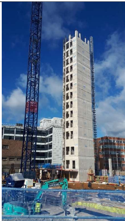
Photo 3 – View facing northwest across site showing Block E construction (north core)
