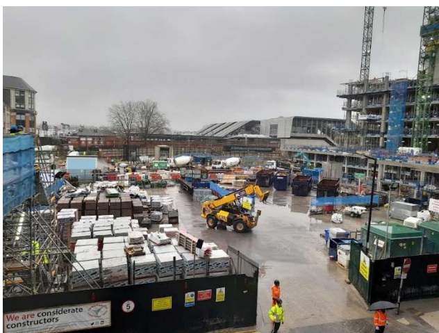
Photo 3 – Combined storage area in Phase 2.
