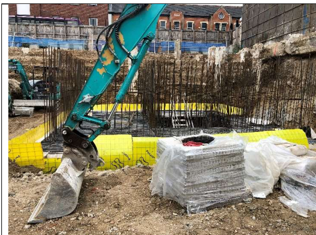
Photo 1 – Block E southern core excavated and installed.
