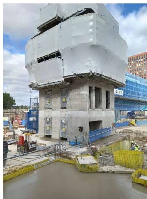
Photo 2 – View of the core construction in the north west of the site.
