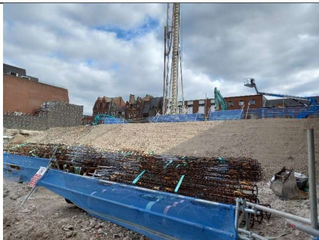
Photo 7 – Southern extent of the site at formation level (excluding south east corner). Piling rig operational.
