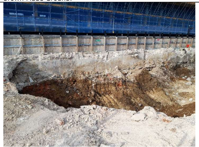
Photo 4 – Cross section view of the northern boundary to the south site. Blue area shows current demolition works of the NCP car park on the north site in the background.
