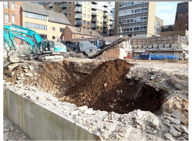
Photo 2 – View facing south east across the excavation in the north east of the south site. Concrete slab overlying brown Made Ground.
