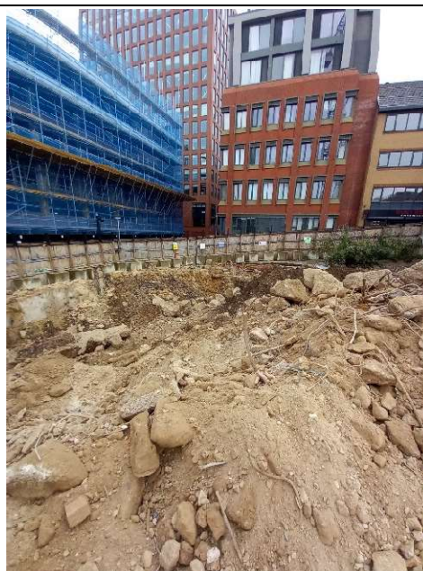
Photo 6 – View of broken out concrete slabs and exposed Made Ground in the northeast of site.
