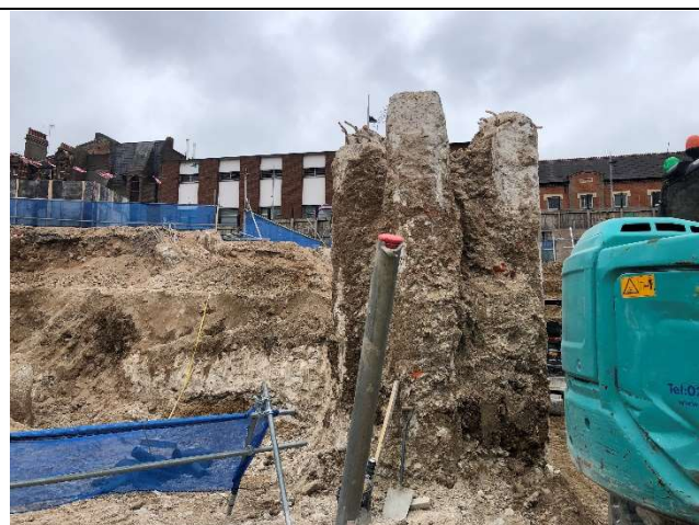
Photo 2 – Exposed piles within southwest of the site.
