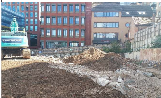
Photo 5 – Concrete boulders and Made Ground in northeast of site awaiting removal for crushing and replacement as piling mat in the northeast and east (for Block F).
