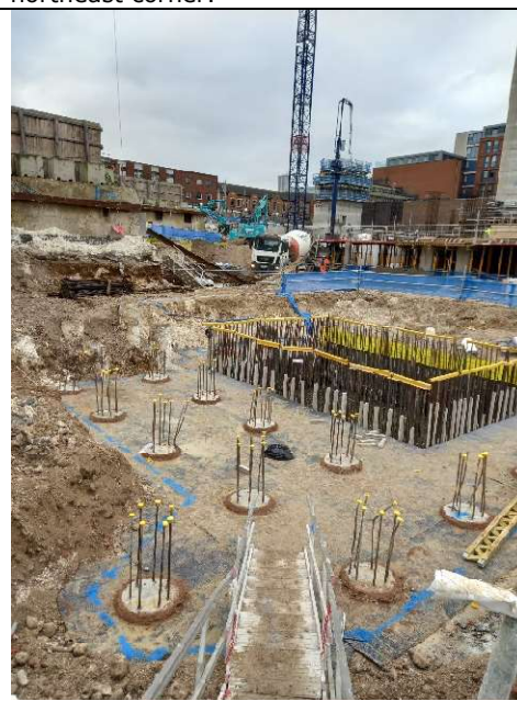
Photo 4 – View of eastern area with pile caps installed.
