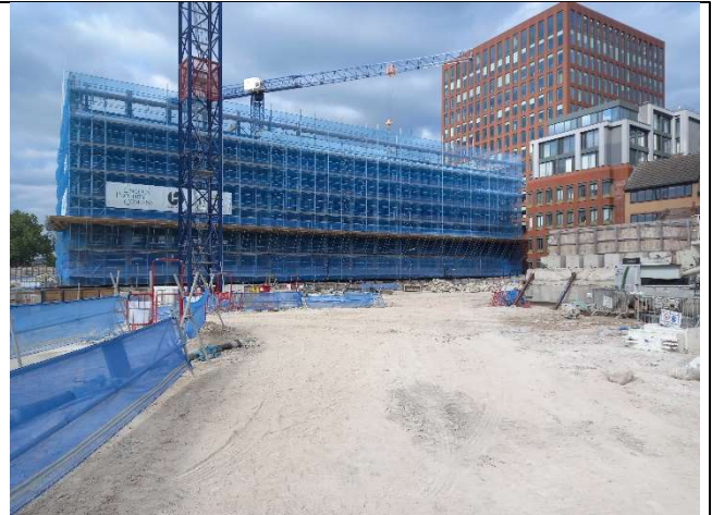
Photo 12 – Concrete slab yet to be removed along the eastern and north eastern extent of the site. Breaking out of the slab has started in the far north east corner of site (see photograph below).
