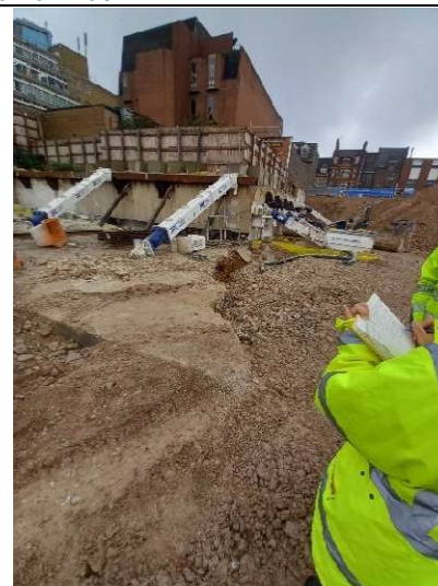
Photo 4 – Last remaining concrete slabs awaiting breaking out in northeast of the site.
