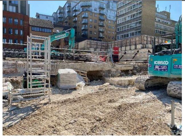
Photo 8 – Close-up view of the concrete slab in place in the north eastern section of the site.
