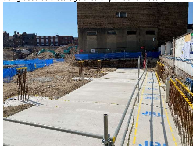
Photo 12 – Concrete slab emplaced in the north west corner of the site. Services are to be installed here.
