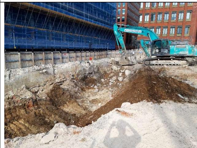
Photo 3 – View of the north eastern boundary of the south site
