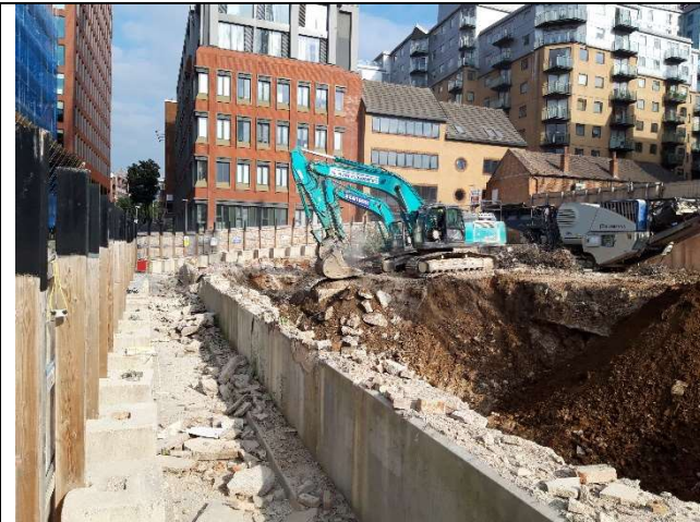
Photo 1 – View facing east across the current excavation in the north east of the south site
