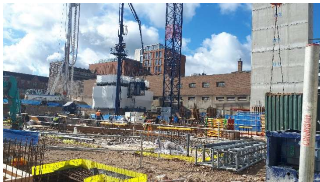
Photo 1 – View facing south west across the site showing construction of Block E.
