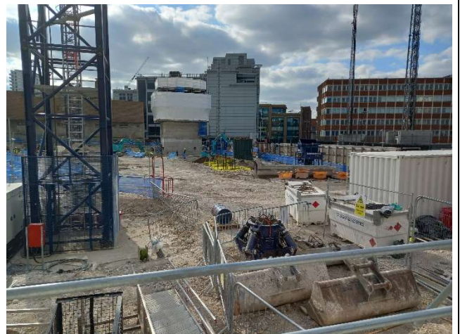
Photo 14 – View facing west across the site.
