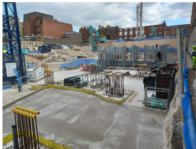
Photo 4 – View along the western site boundary. Concrete slab progressed.
