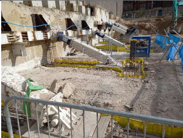
Photo 11 – View of the retaining wall on the eastern site boundary. New steel supports emplaced upon support piles.
