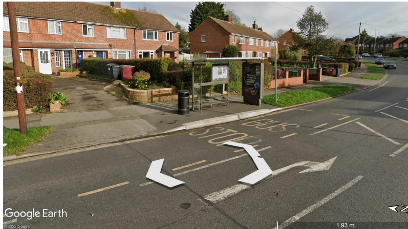
Figure 3.5: Existing bus shelter on Southcote Road (near Frilsham Road junction)
