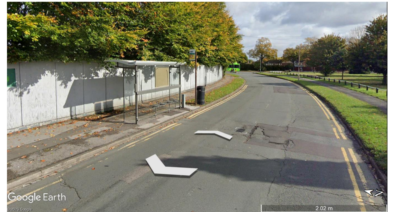
Figure 3.2: Existing bus shelter on Dwyer Road (site frontage)
