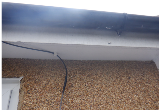
9. Soffit tight to rendered wall (south elevation).
