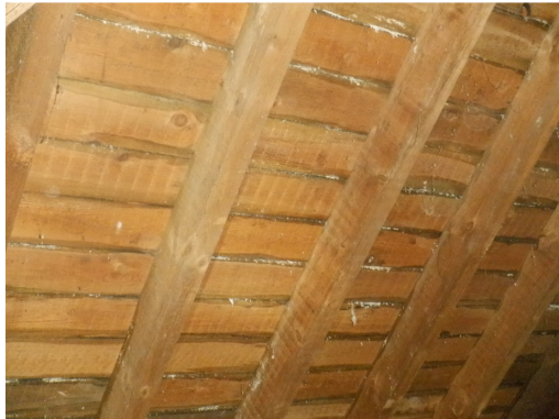
13. Intact timber sarking (roof void).
