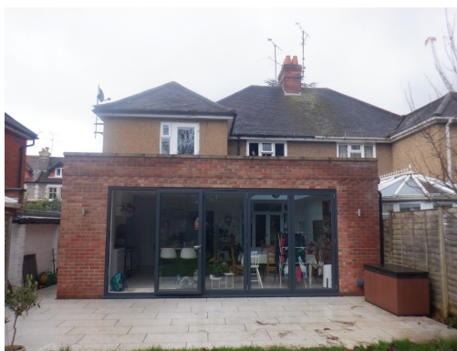
2. Rear of property viewed from south.
