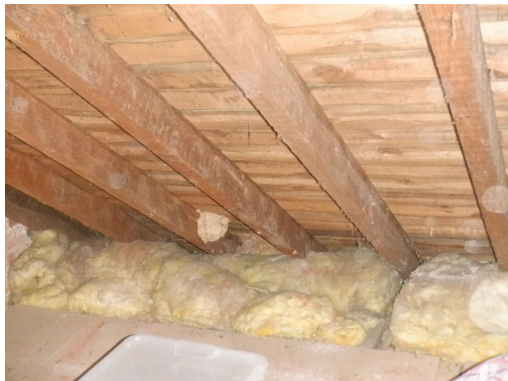
17. Part open eaves (roof void).
