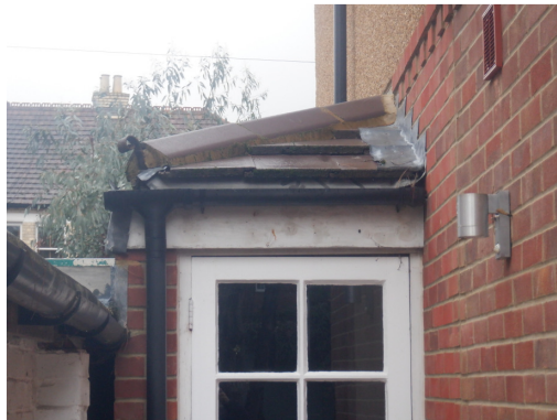
10. Intact hip mortar and flat roof tiles (rear elevation).
