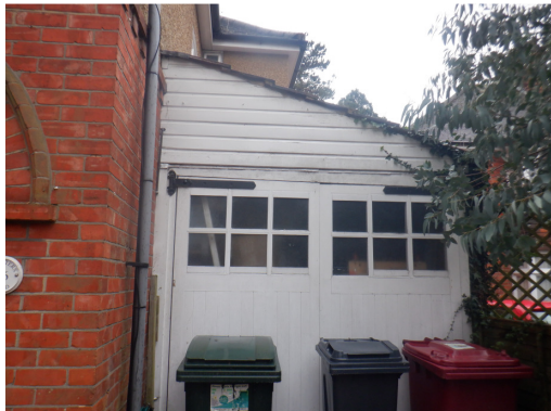
11. Tight timber cladding on garage (front elevation).
