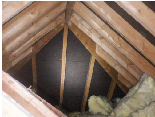
14. Intact hessian reinforced bitumen felt (roof void).
