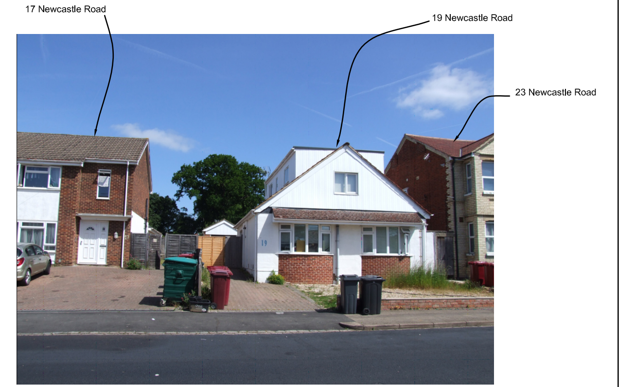
Existing Street Scene Photograph showing 17, 19 and 23 Newcastle Road
