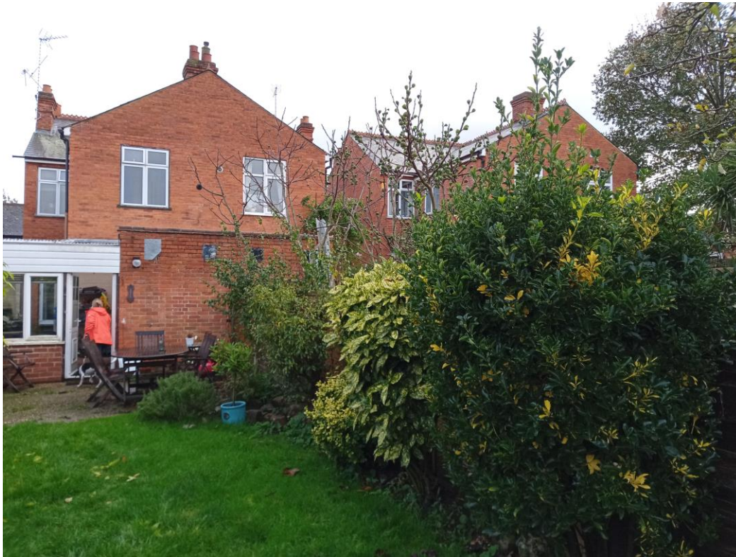
Figure 2: 26 & 28 Clifton Street - Existing Rear (site visit 16/11/2022)
