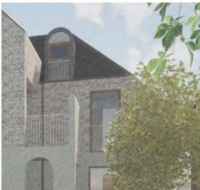
South facing terrace to apartment 04 with arched lintel details and dormers
