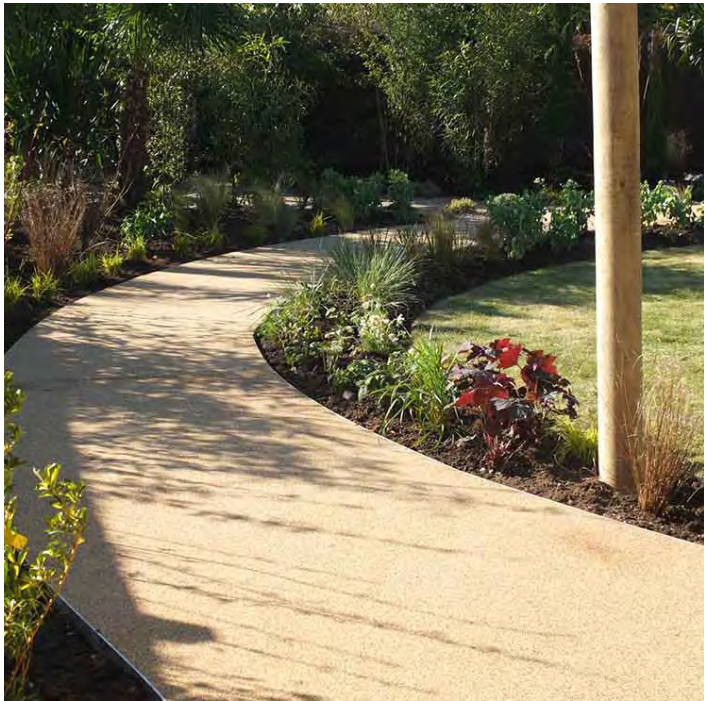
Resin bound gravel paths to the respite facility garden with metal edging
