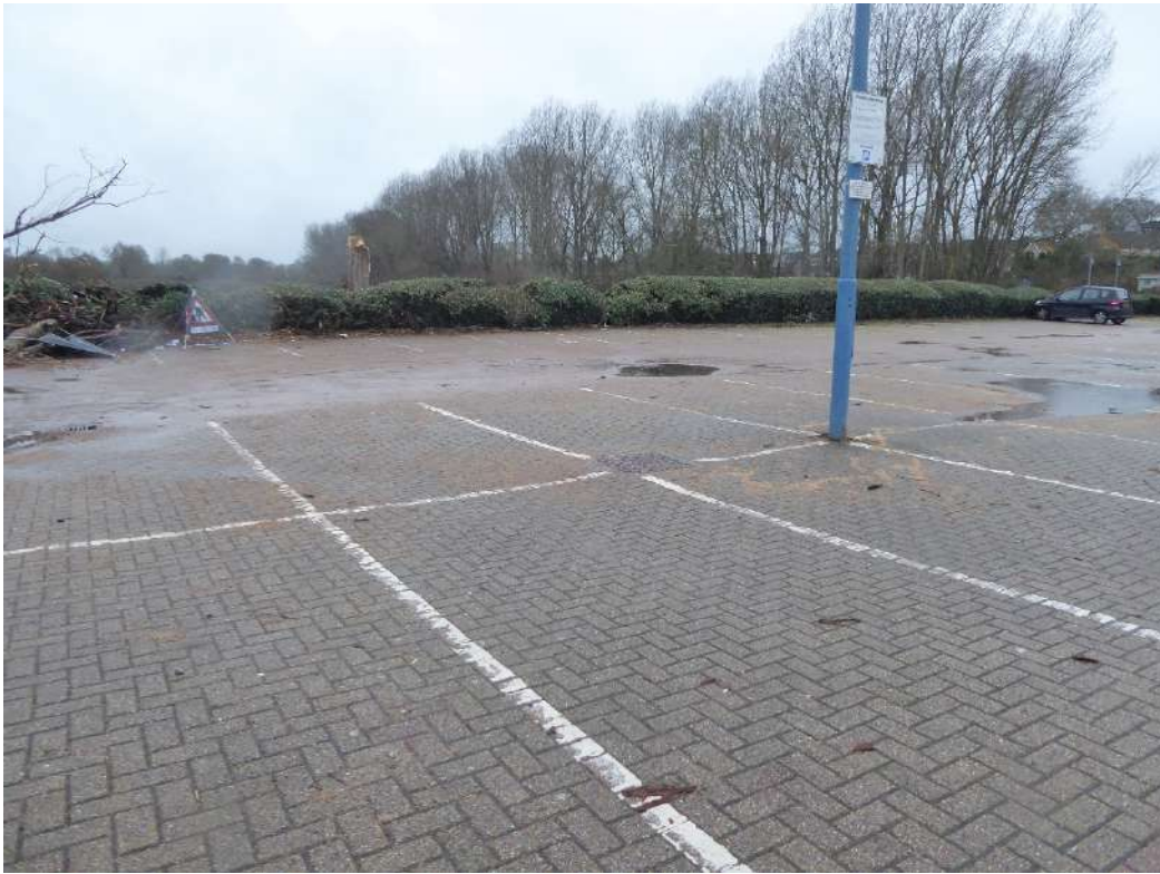
DP 5. View north-westwards across the Site, which comprises hardstanding carparking consisting of two rows of car parking spaces.
