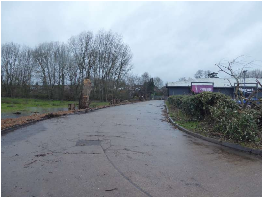
DP 9. View northwards of the service road for delivery and refuse vehicles to the Reading Link Retail Park, which lies to the immediate west of the Site
