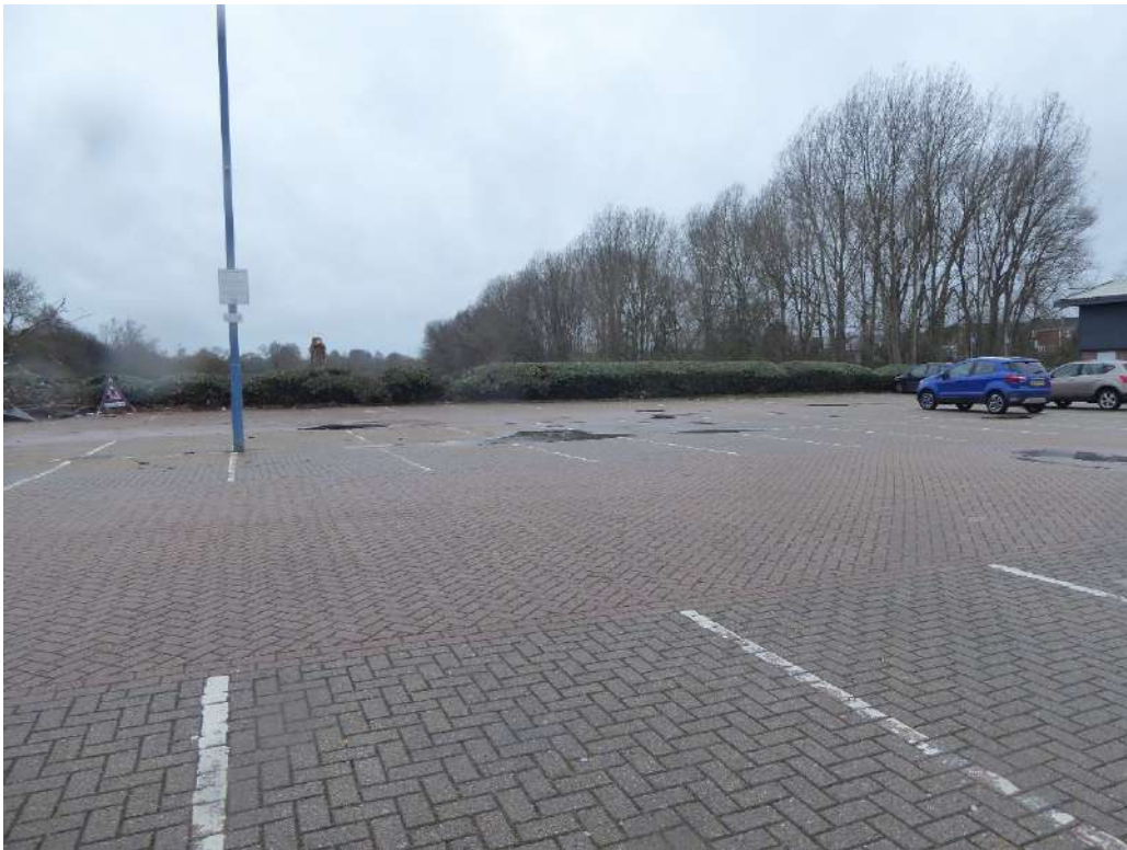
DP 7. View westwards across the Site, which comprises hardstanding carparking consisting of two rows of car parking spaces.
