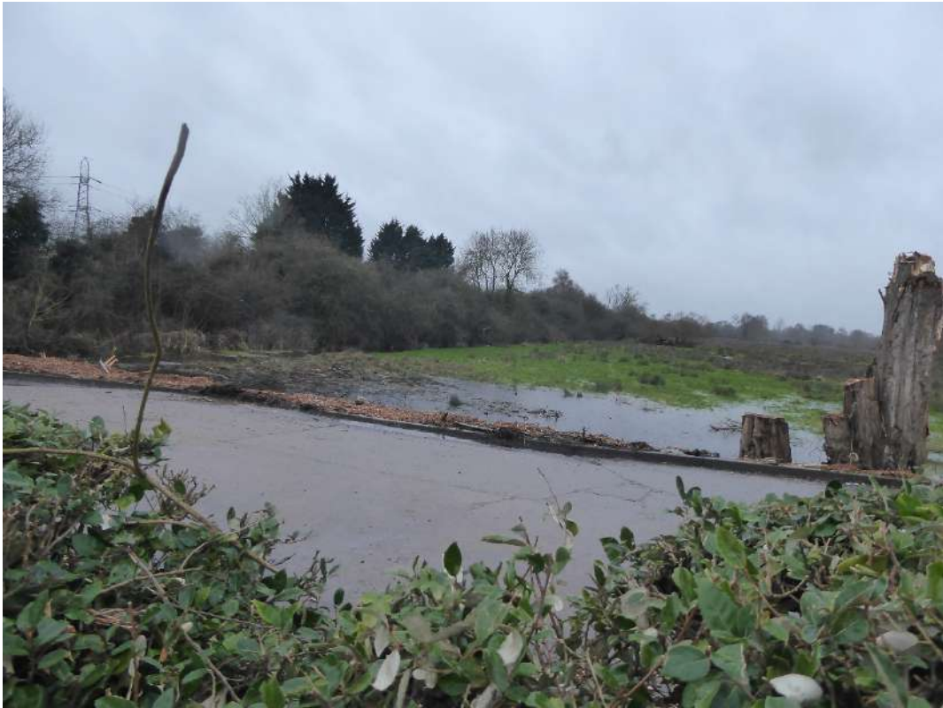
DP 3. View south-westwards of the services road and lower-lying floodplain, both of which lies to the south-west of the Site.
