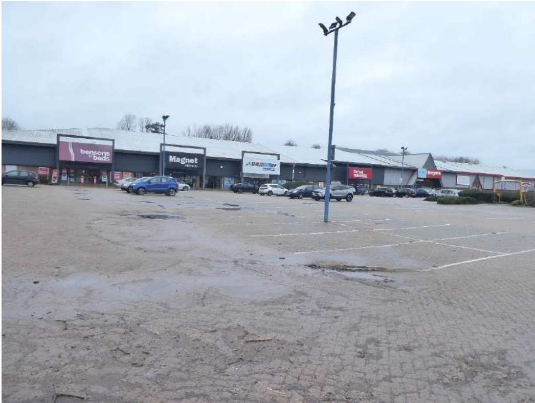
DP 1. View northwards of the Reading Link Retail Park from the south and across the associated hardstanding car park, which includes the Site.
