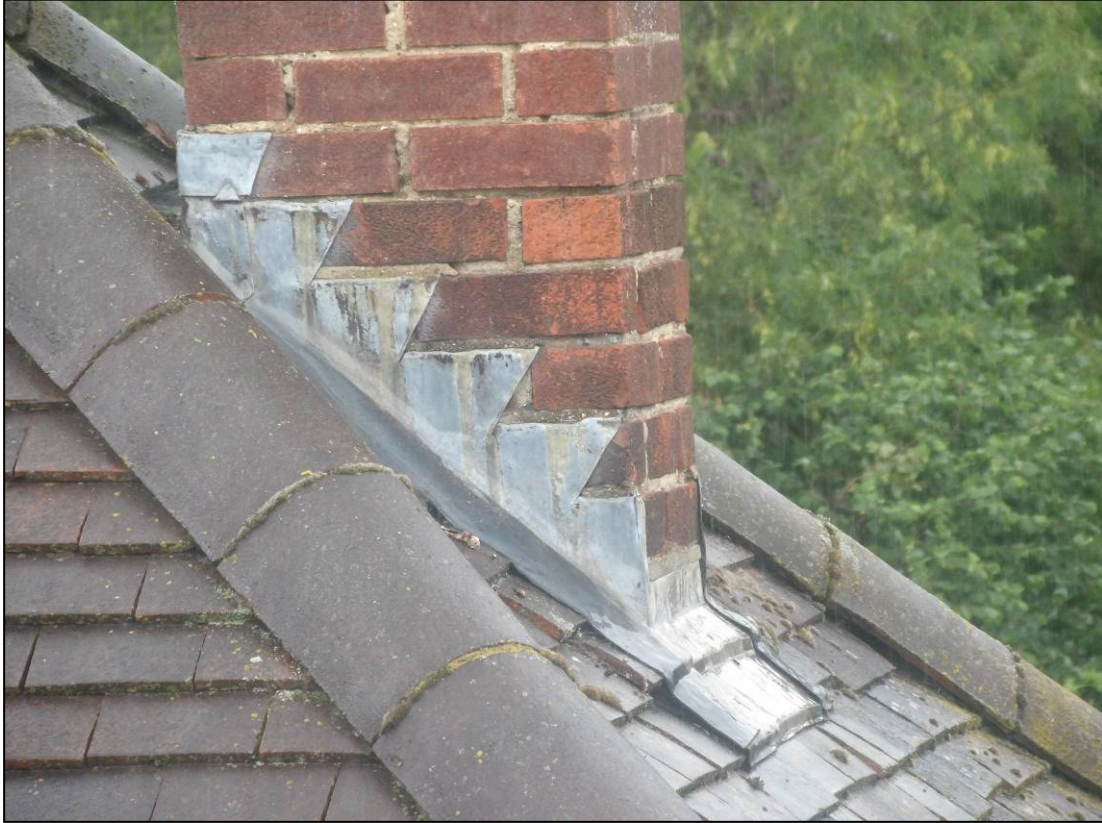
Figure 7. Lead flashing around the chimney. 10 Courtenay Drive, Emmer Green. 04.07.23
