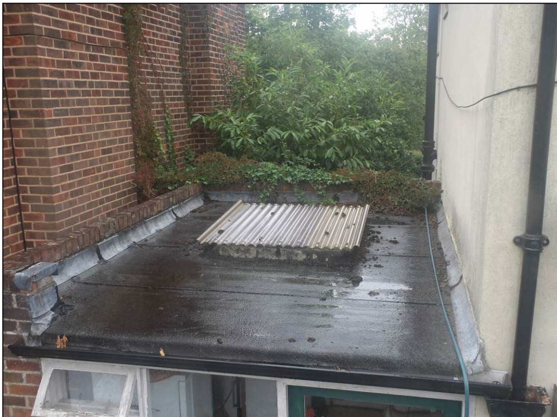
Figure 10. Roof of single storey extension. 10 Courtenay Drive, Emmer Green. 04.07.23
