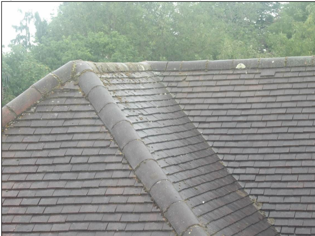
Figure 6. Example of ridge and hip tiles. 10 Courtenay Drive, Emmer Green. 04.07.23
