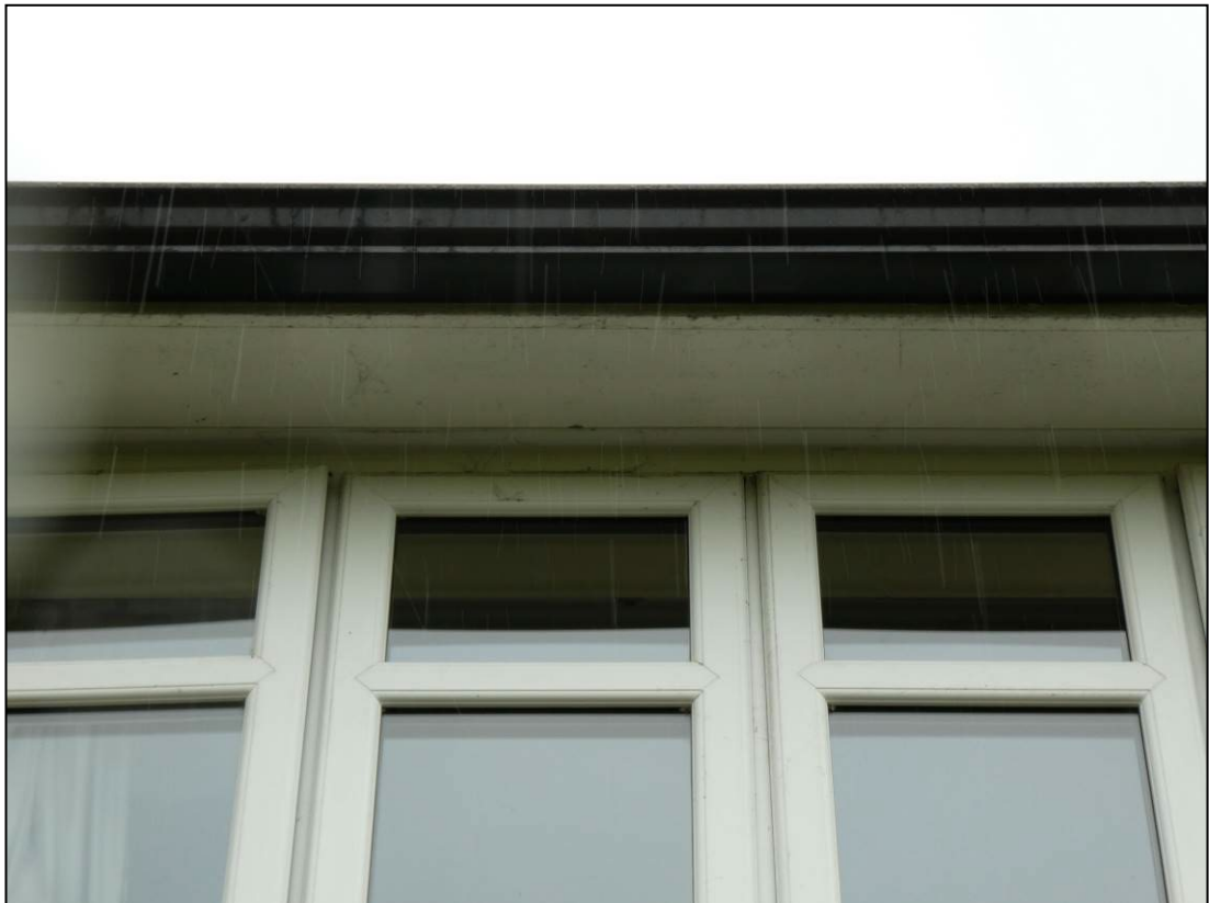
Figure 8. Soffits and fascia's. 10 Courtenay Drive, Emmer Green. 04.07.23
