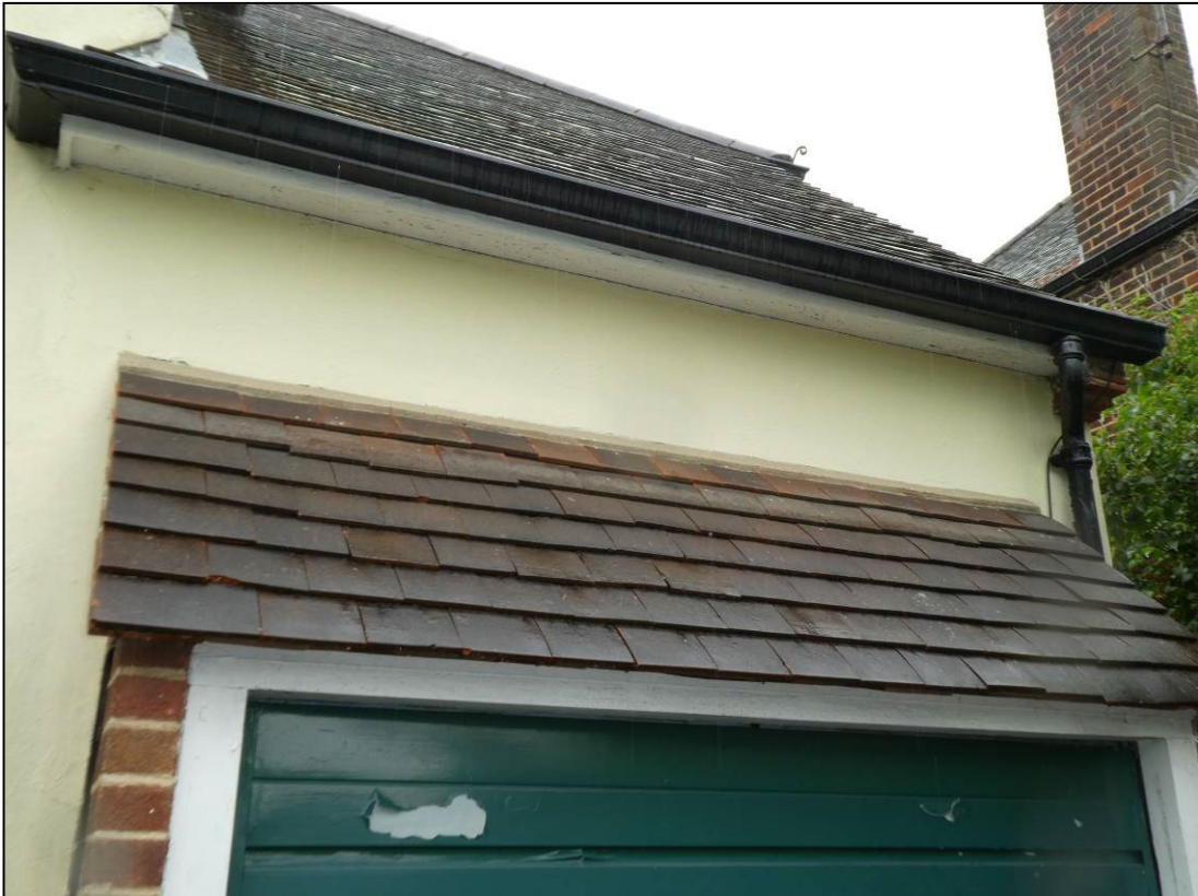
Figure 12. Roof of integral garage. 10 Courtenay Drive, Emmer Green. 04.07.23
