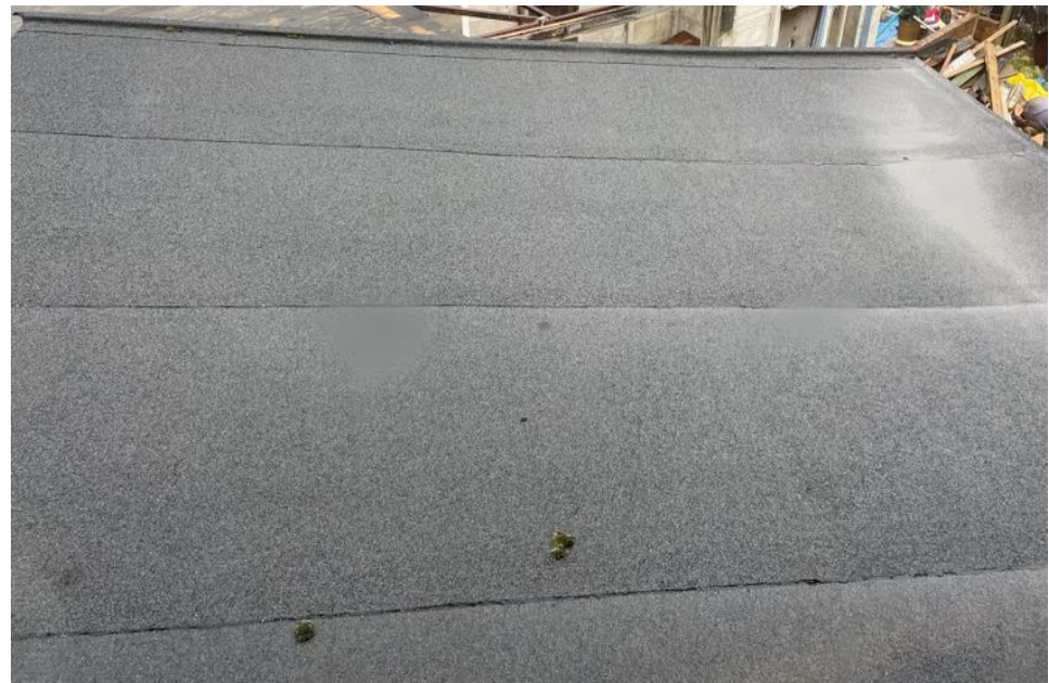
Figure 4: the flat roof of B2
