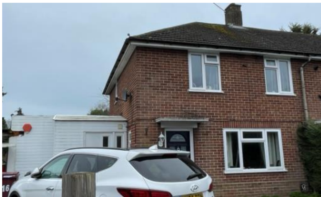
Figure 1: the northern elevation of B1 and B2
