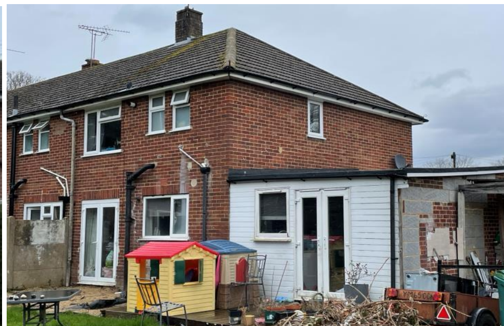
Figure 2: the eastern and southern elevations of B1 and B2
