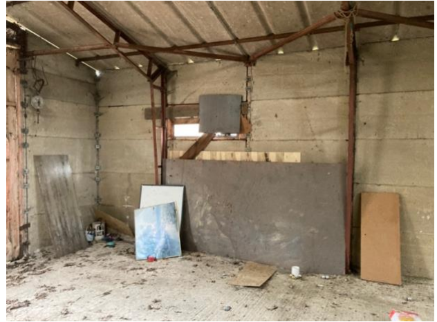
Photograph 8: Interior of building
