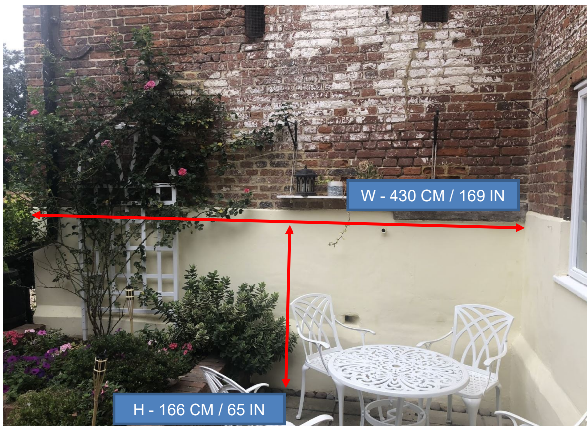
Fig 0B:East-facing adjoining wall ext masonry
