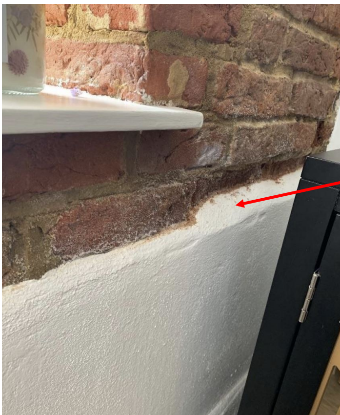
Fig 0D: Int masonry 2 of 2
