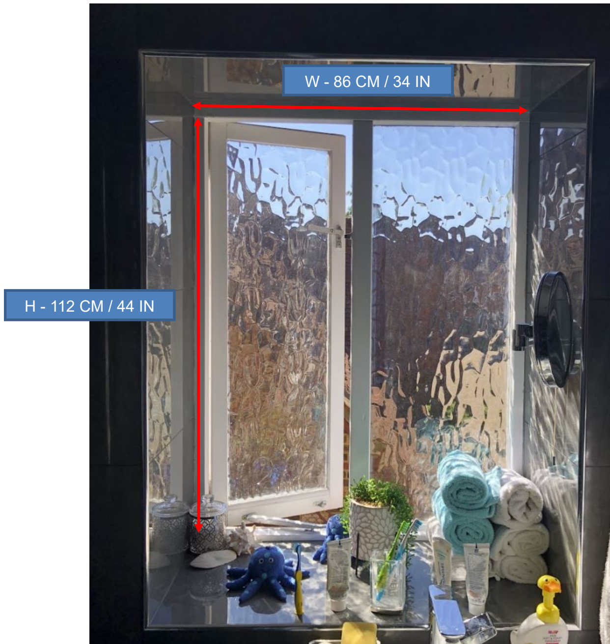
Fig 6C:Scale-drawing proposed replacement Window Six, south-facing bathroom window with annotations(int)
