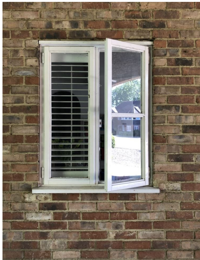
Fig 1B:Window One, west-facing lounge window(ext)
