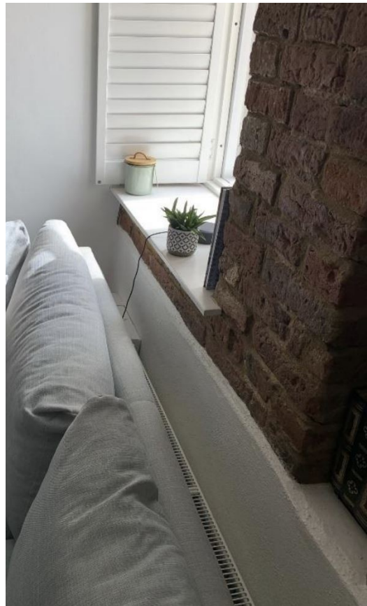
Fig 0C: Int masonry 1 of 2
