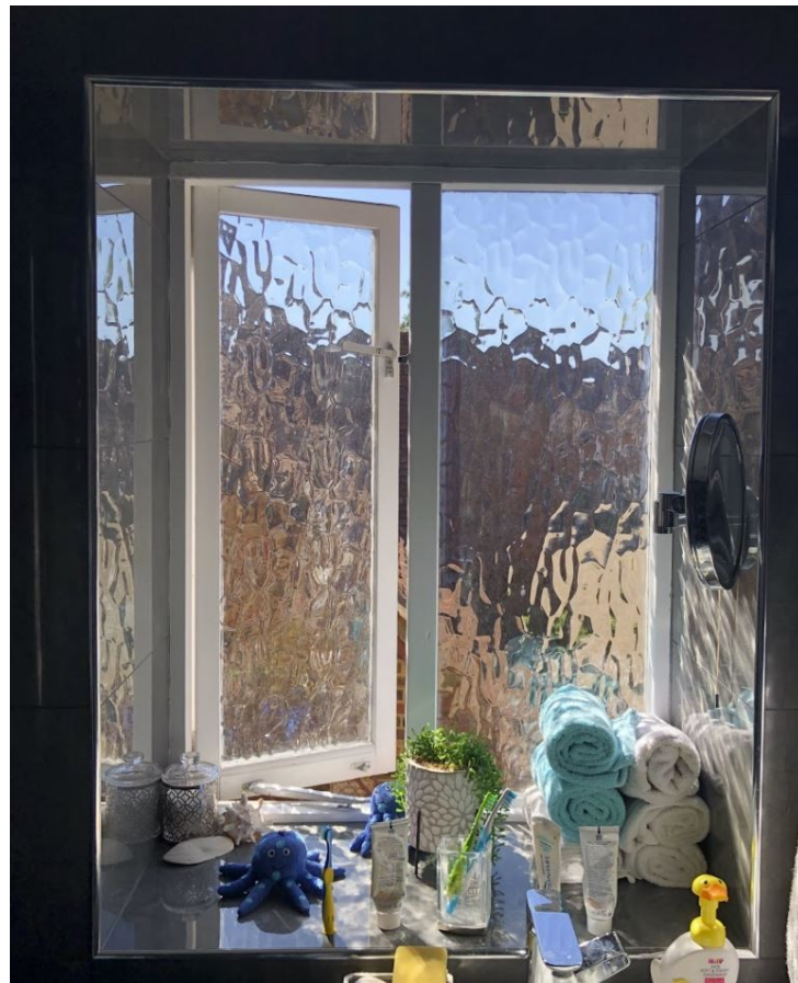
Fig 6A:Window Six, south-facing bathroom window(int)
