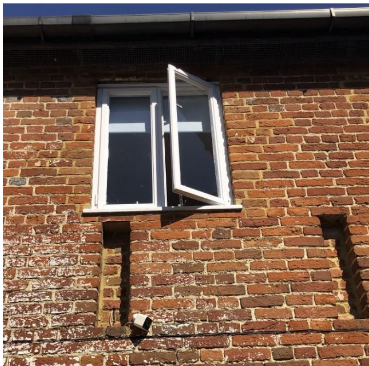
Fig 5B:Window Five, south-facing first bedroom window 2 of 2(ext)
