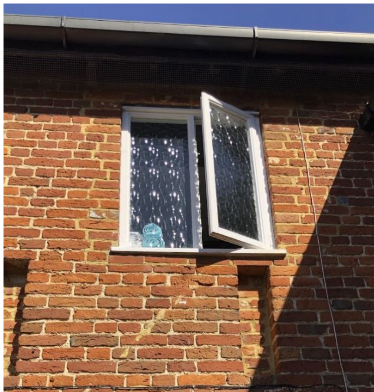
Fig 6B:Window Six, south-facing bathroom window(ext)
