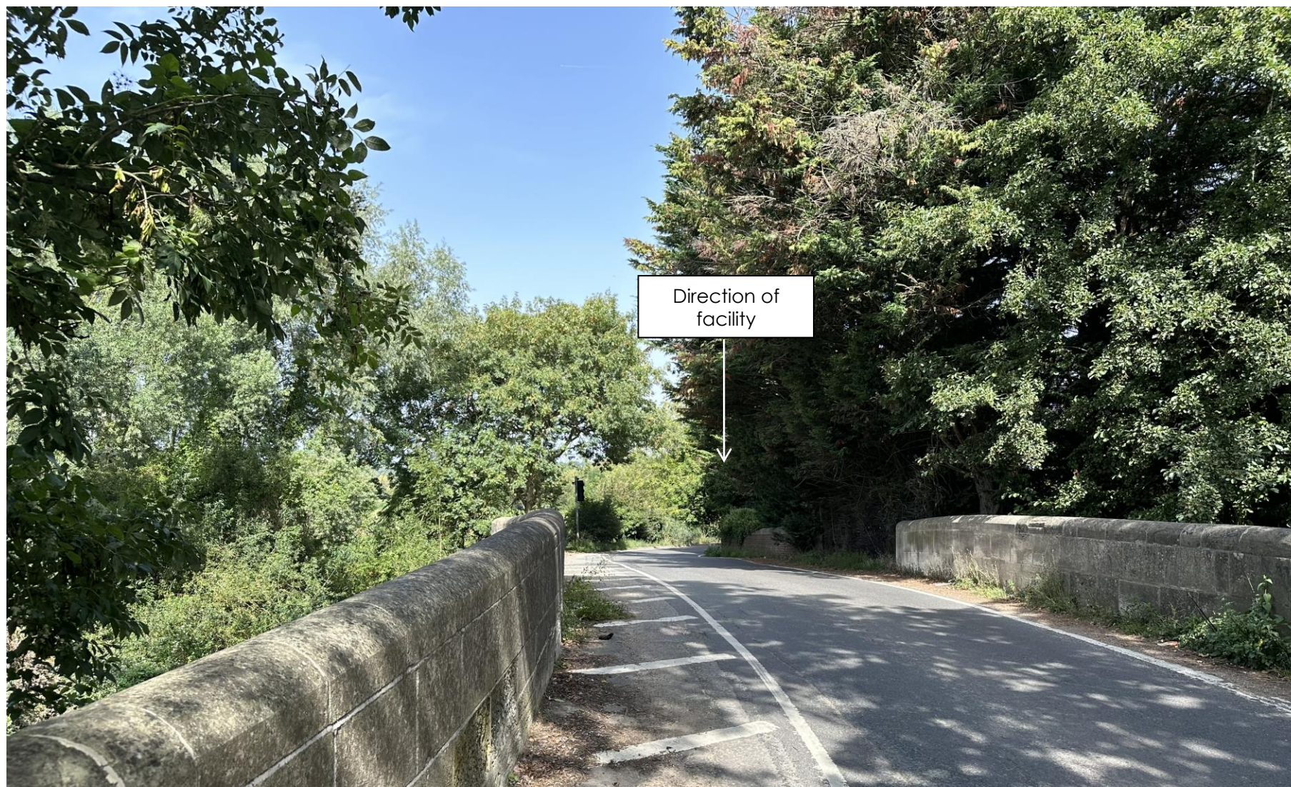
View 9 From Burghfield Bridge south of site.
