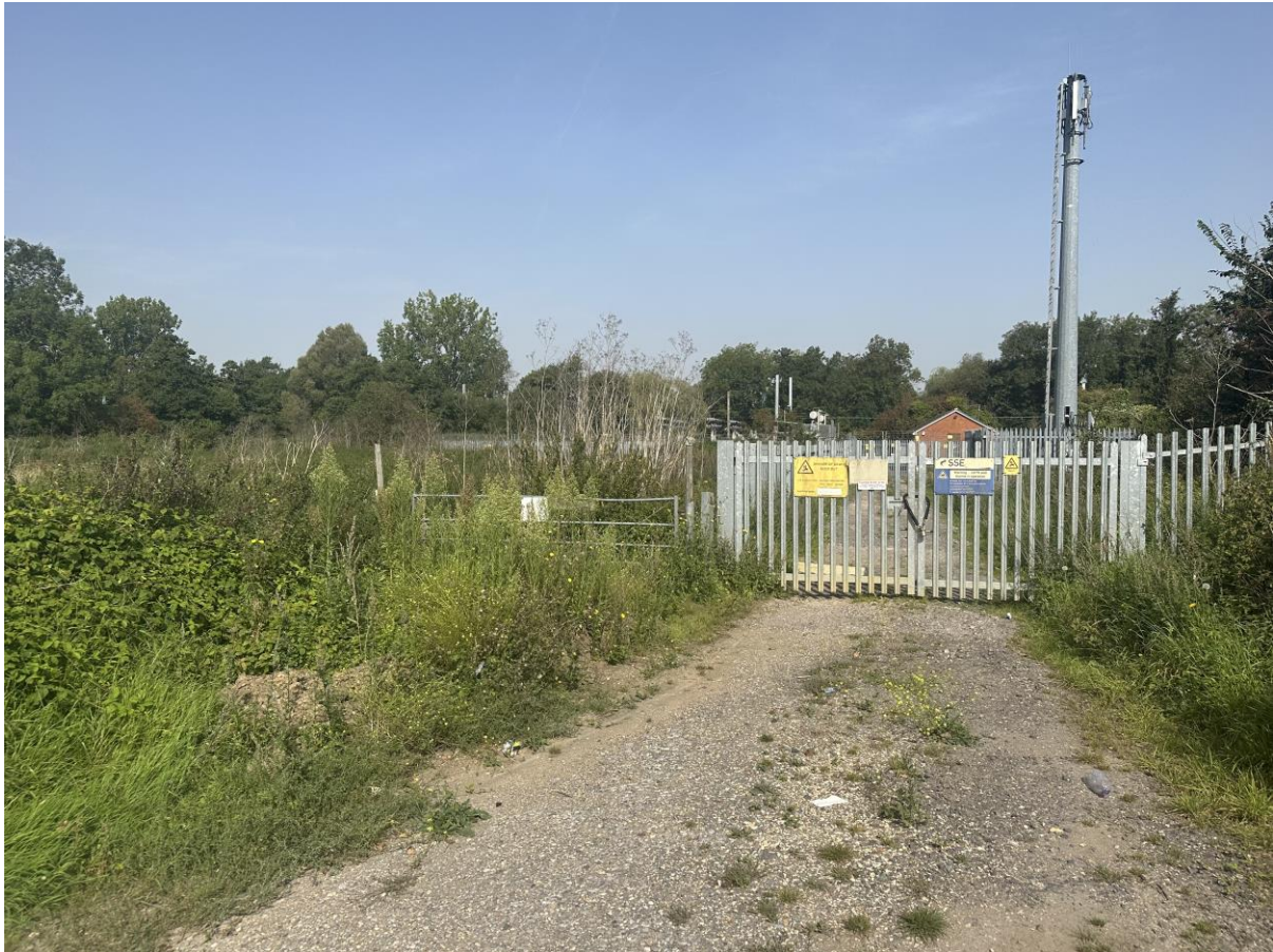
Existing access track to sub-station
