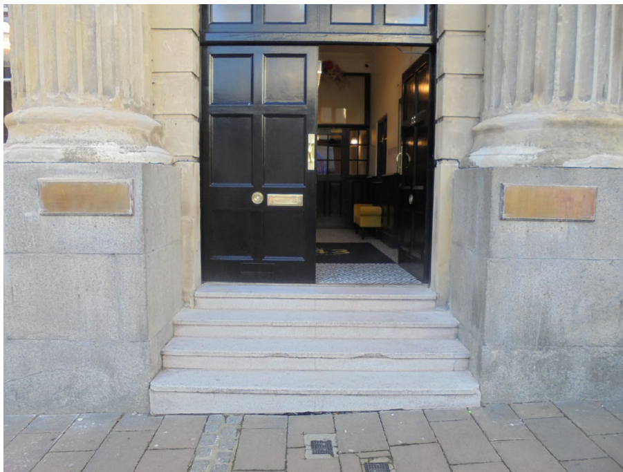
Photo 2 and 3– Close up view of the entrance
