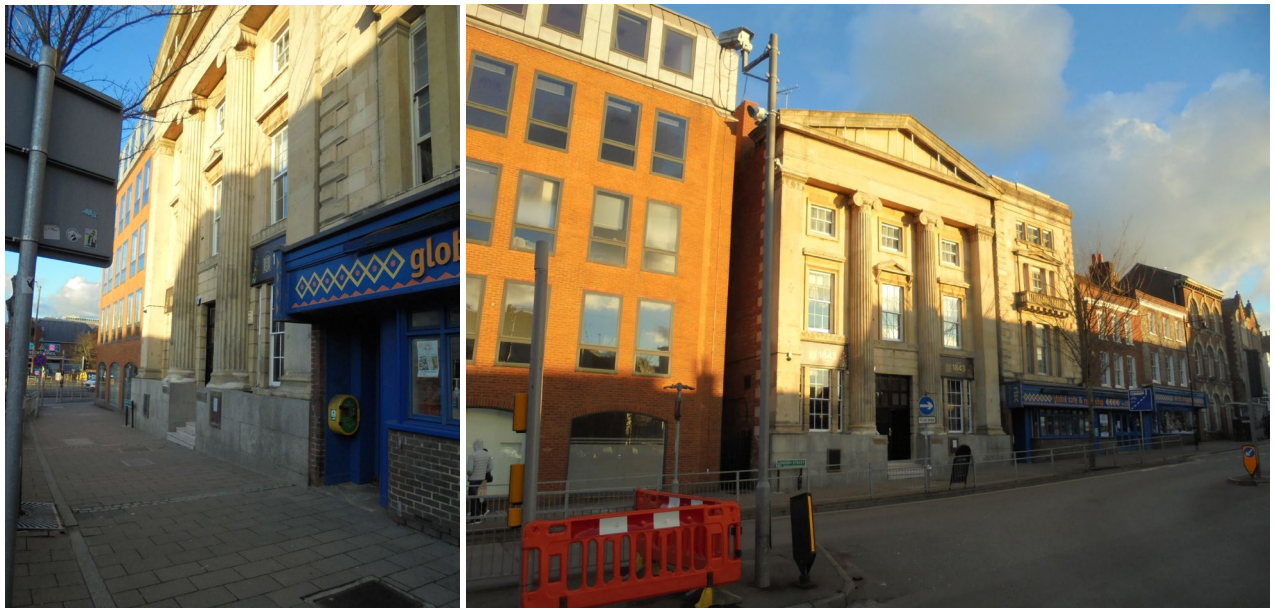
Photo 5 and 6 – Streetview of the property and it's proximity to other Listed buildings
