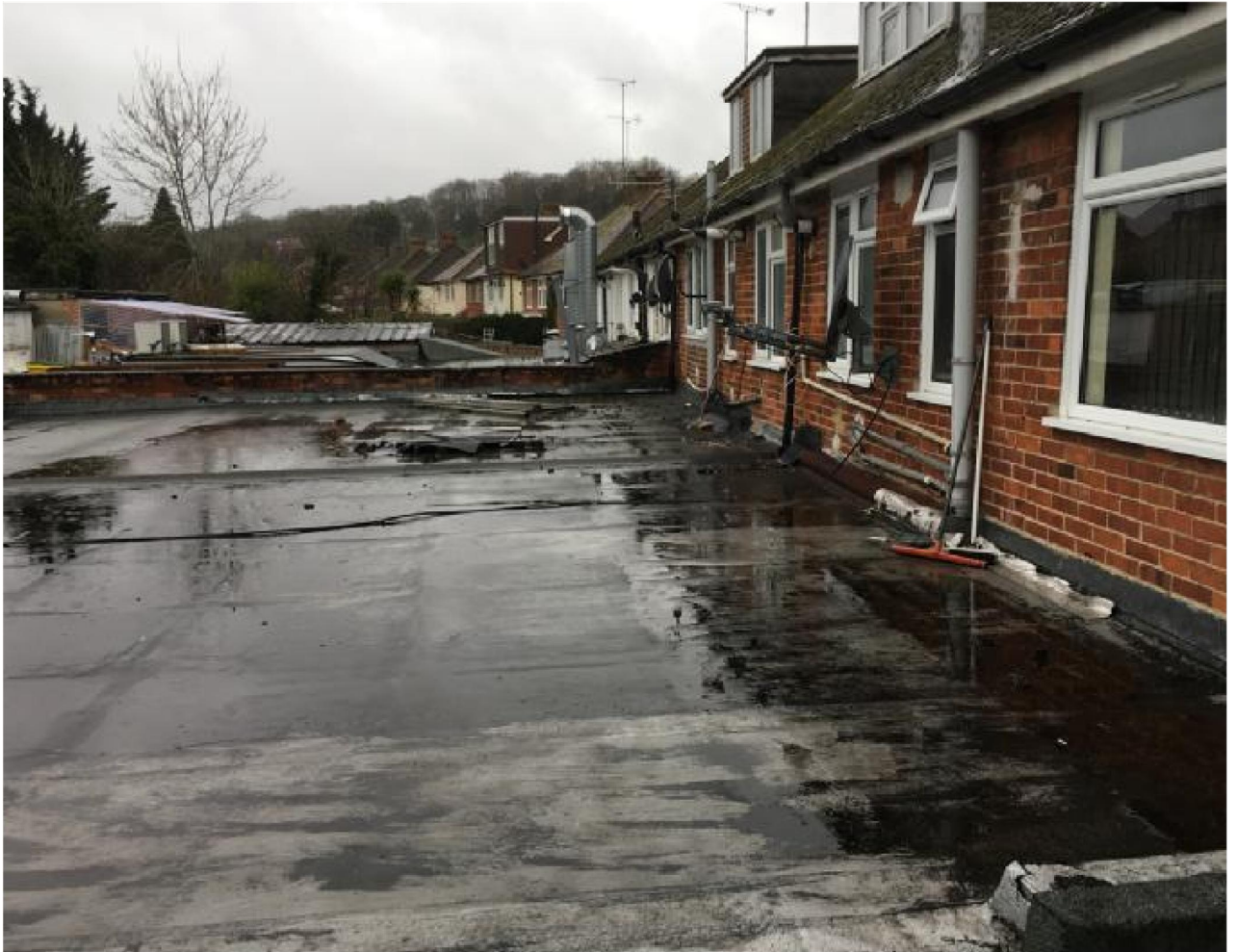
Figure 5 Rear of Costcutter Continued.
