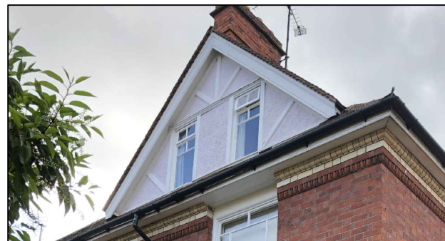
Existing third floor windows of No.6 The Mount are set within rough cast render and exposed timber frame painted white
