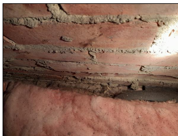
Photo 10 Floor at base of gable apex
