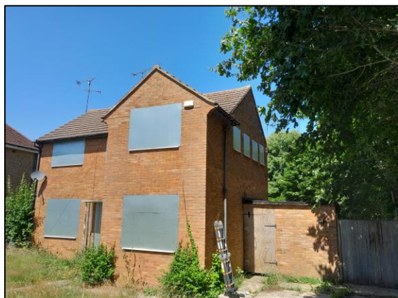
Photo 1 Front (south) elevation and east side elevation, showing flat roof extension
