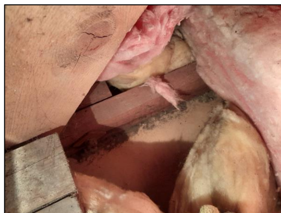
Photo 6 Spot checks under insulation
