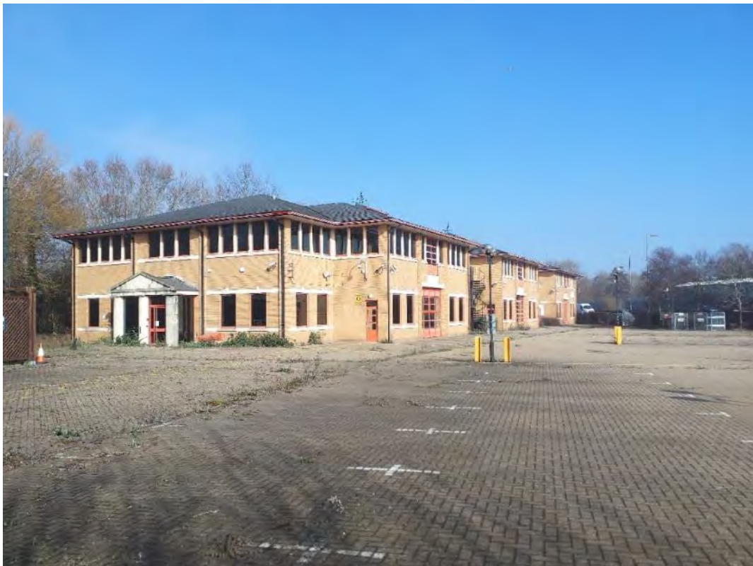
Photograph 3 - Main office building and sealed surface
