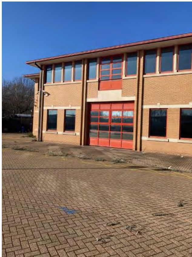
Photograph 1 - Main office building, southern aspect
