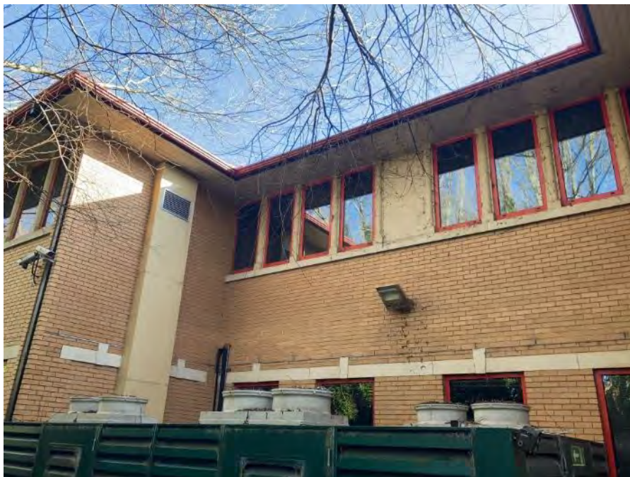
Photograph 2 - Main office building, northern aspect
