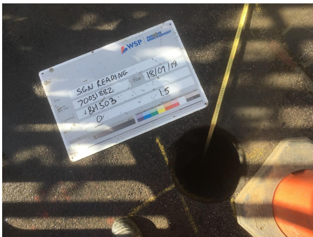
9. BH303: Vacuum excavation hole to 1.5m bgl
