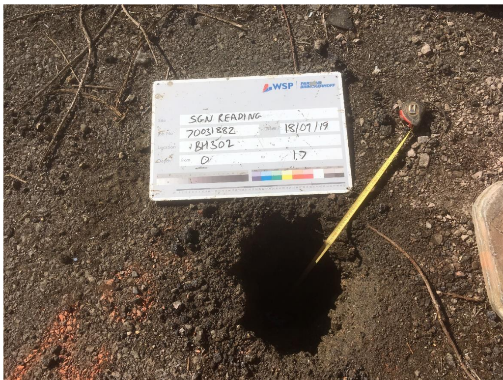
5. BH302: Vacuum excavation hole to 1.7m bgl
